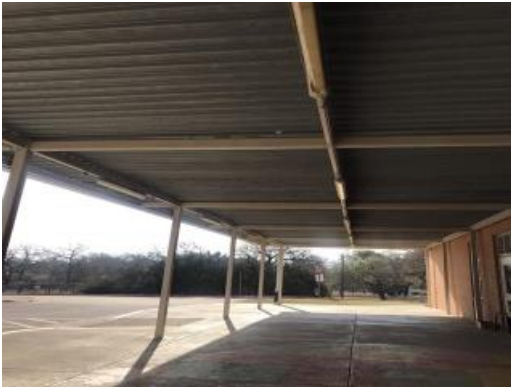
Canopy for outside area
