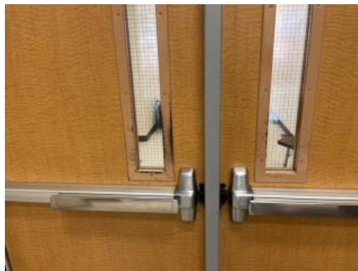
Rusting metal window frame
