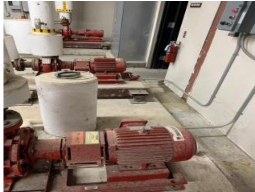
Corroding pumps
