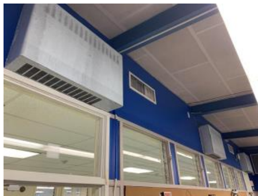
Typical unit ventilator
