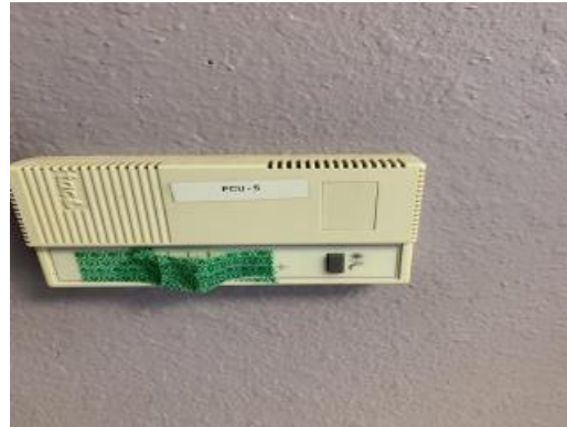
Damaged thermostat
