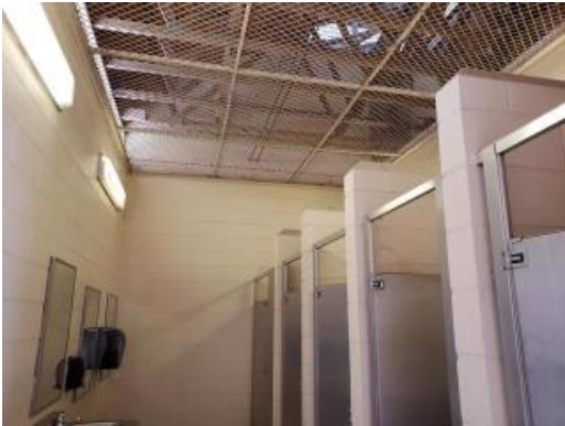
Exposed restroom ceiling
