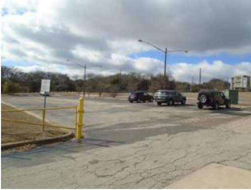
Parking lot pavement
