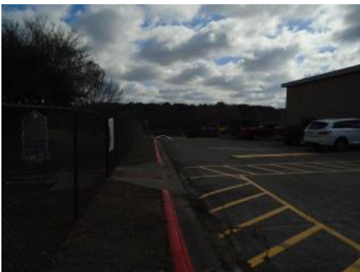
Parking lot asphalt pavement
