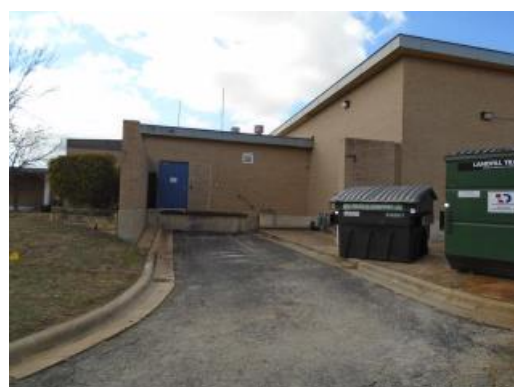
Loading dock pavement
