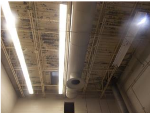
Corroded decking
