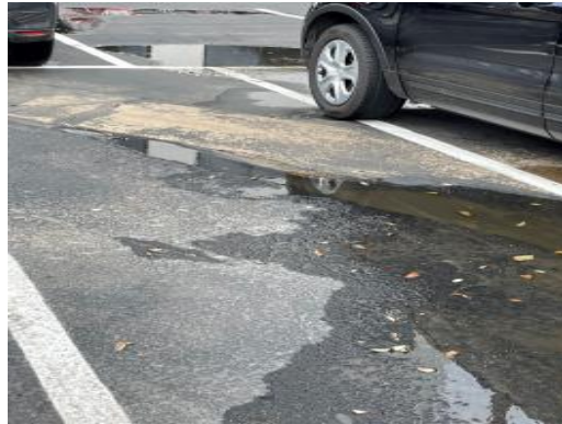
Ponding Asphalt
