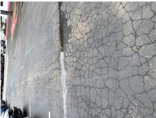
Damaged asphalt
