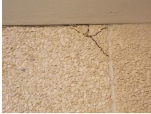
Cracked flooring
