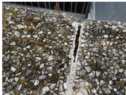
Failed sealant
