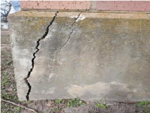
Cracked foundation
