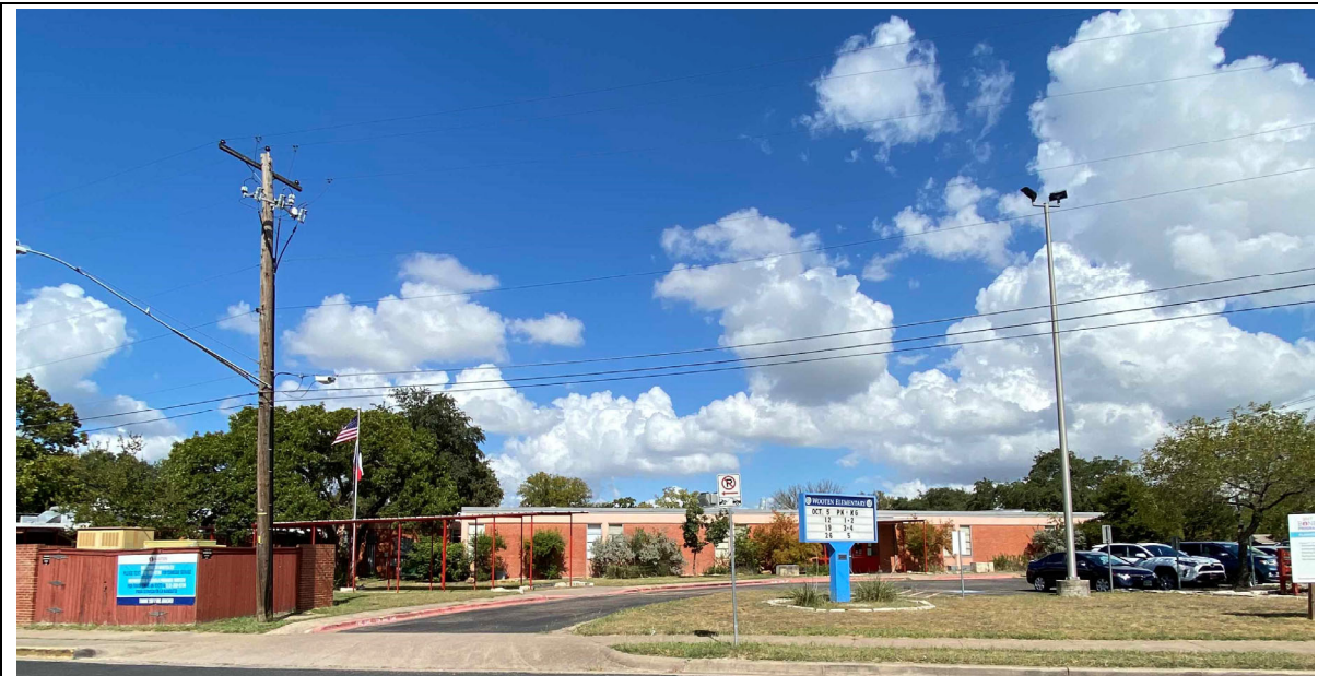
Confusing front entry and flow for visitors into building. Front entry is not where drive is. The school has attempted to make the front entry more visible with plants and signage. Stack space lacking for traffic with student pickup/drop-off on public street.
