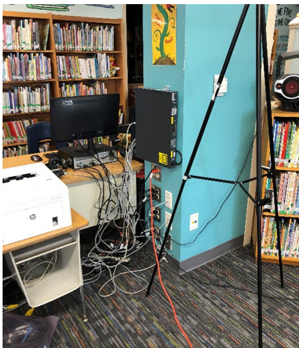
Library (left) and typical studio (right) show outlet connections not dispersed well within spaces.
