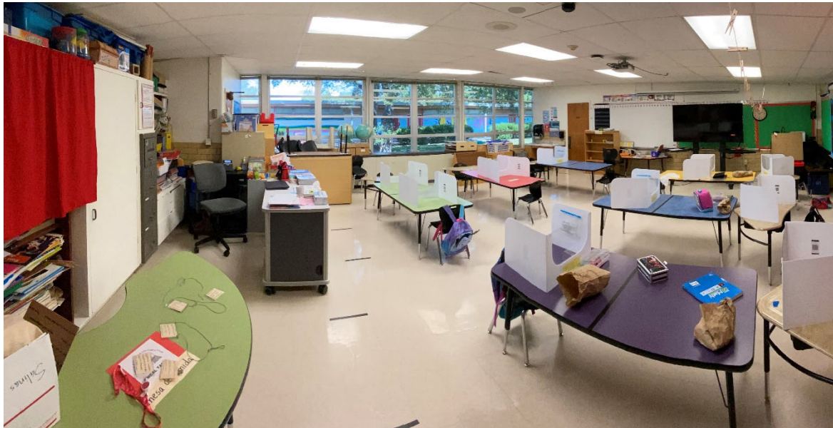
Typical studio has ample daylight. Finishes are dated. Storage is inconsistent between studios and larger tables do not allow for flexible teaching configurations.
