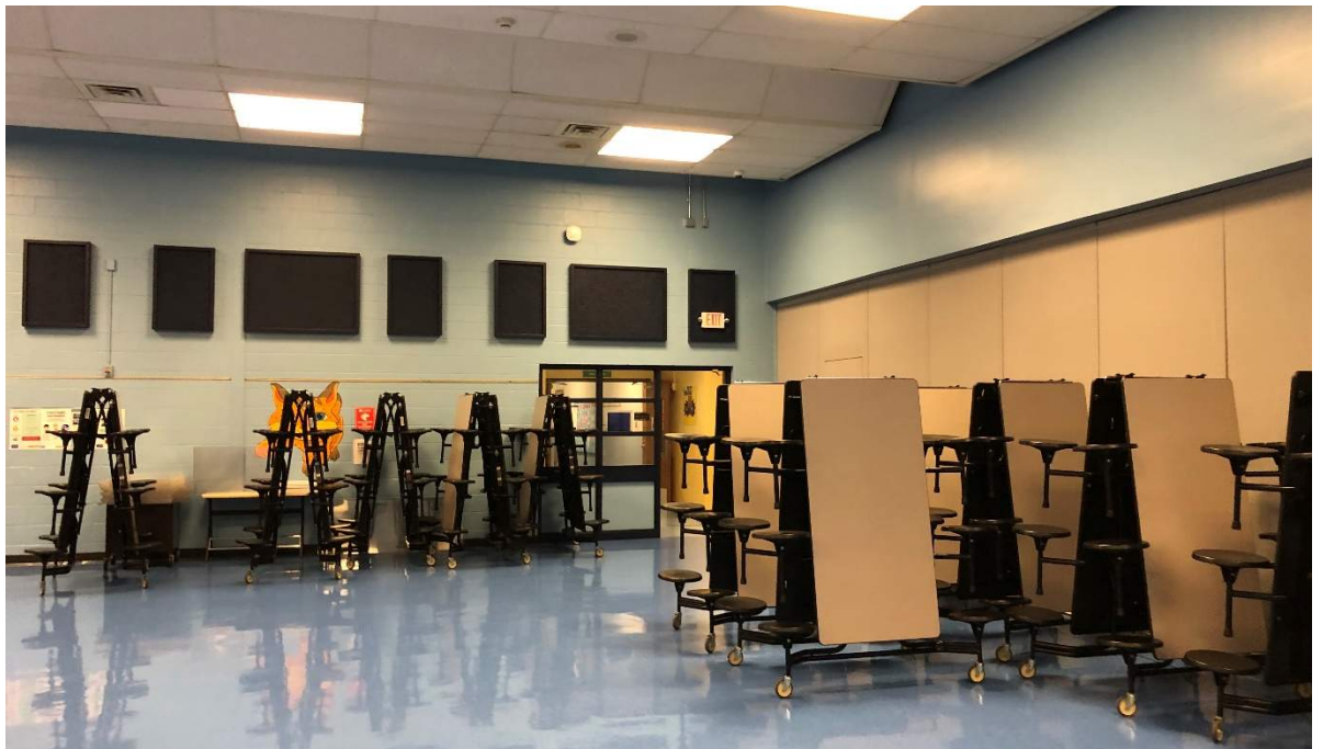
Food Services: Cafeteria is undersized for current school capacity. Stage requires updates, and finishes are dated.
