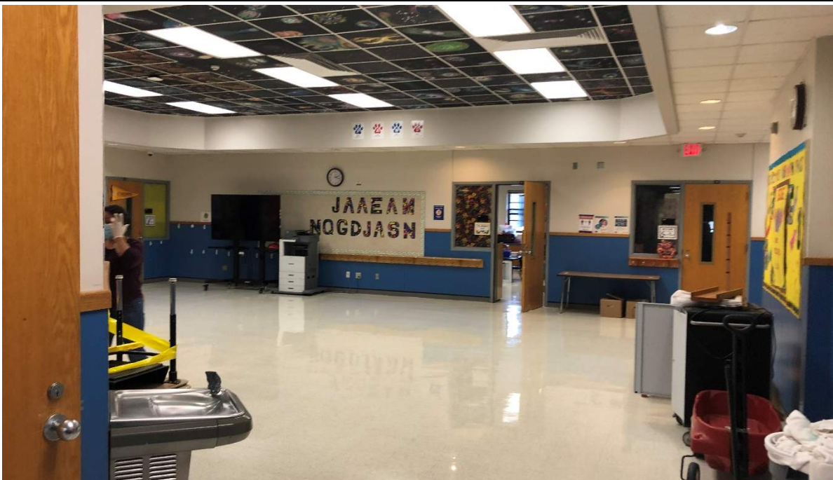
Kindergarten and pre-K wing learning neighborhood with shared common/collaboration space. Studios are connected through a restroom corridor.
