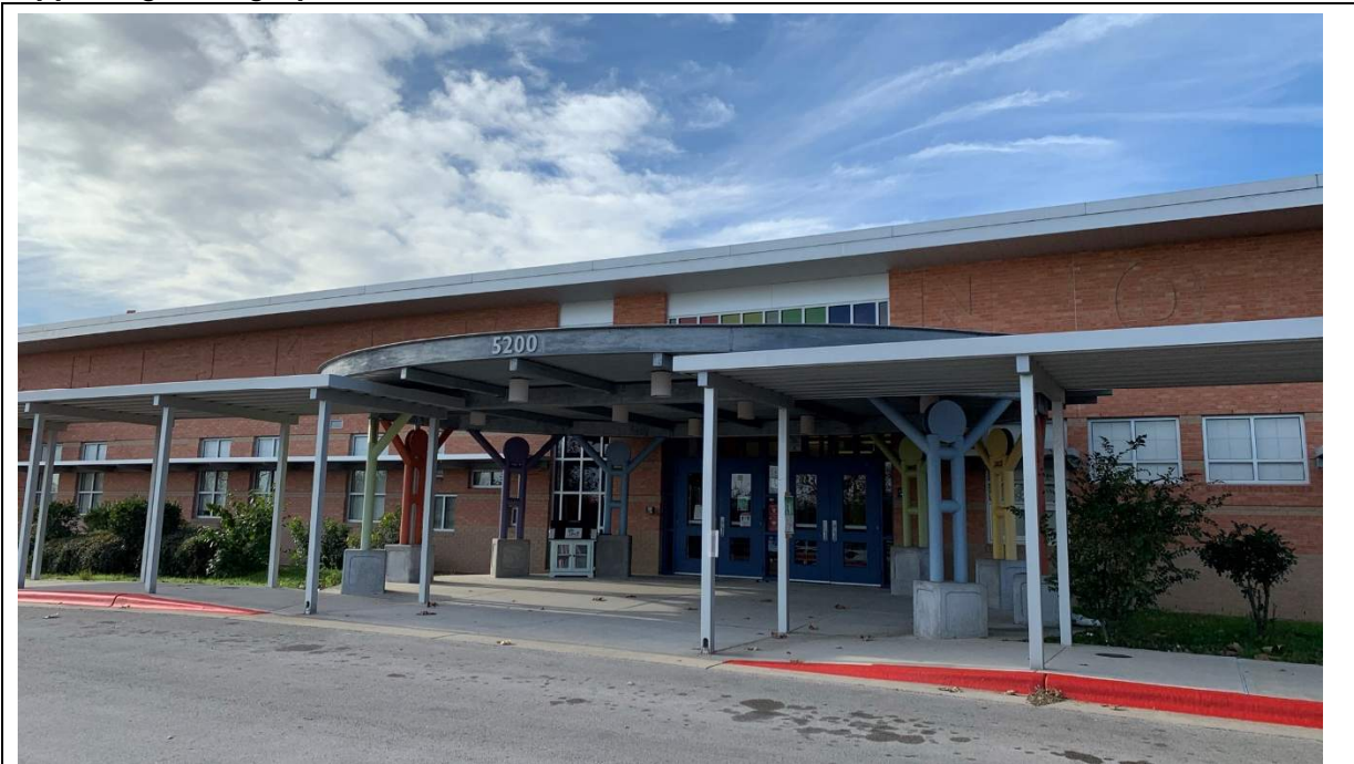
Exterior: Covered main entry and canopy along drop-off area at front of the building.
