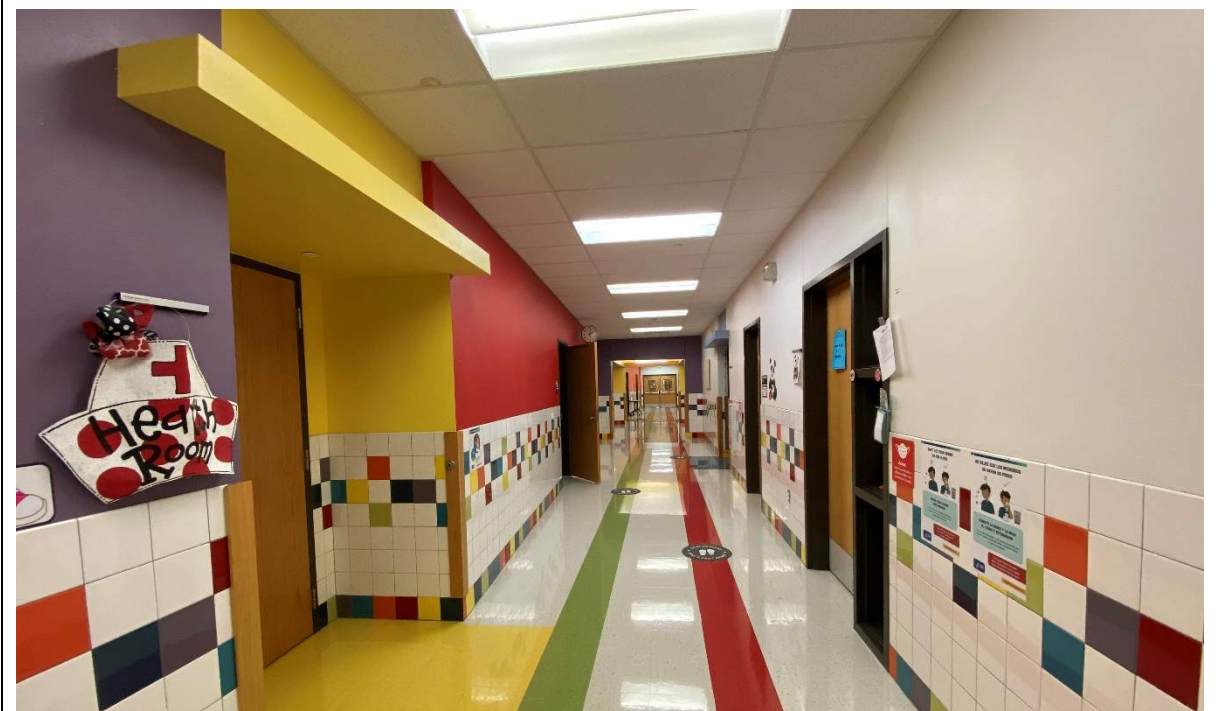
General Building: Corridors vary in width throughout the building, but wayfinding is clarified with colors.
