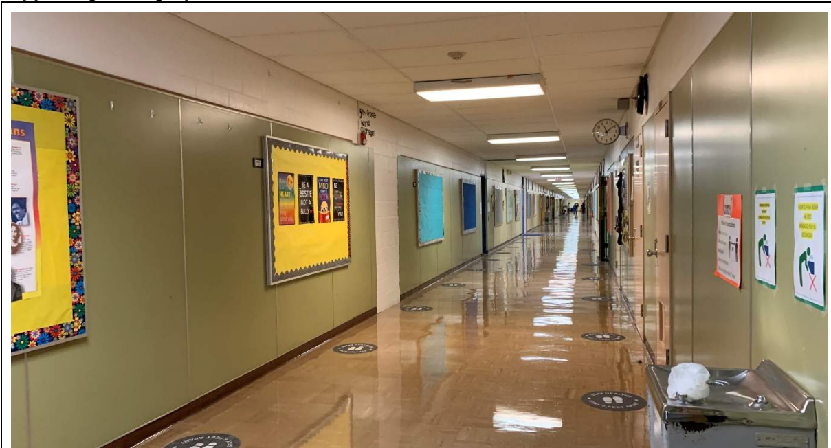
General Building: Main corridor is wide and have ample locations for 2-D display. Finishes and lighting are dated.
