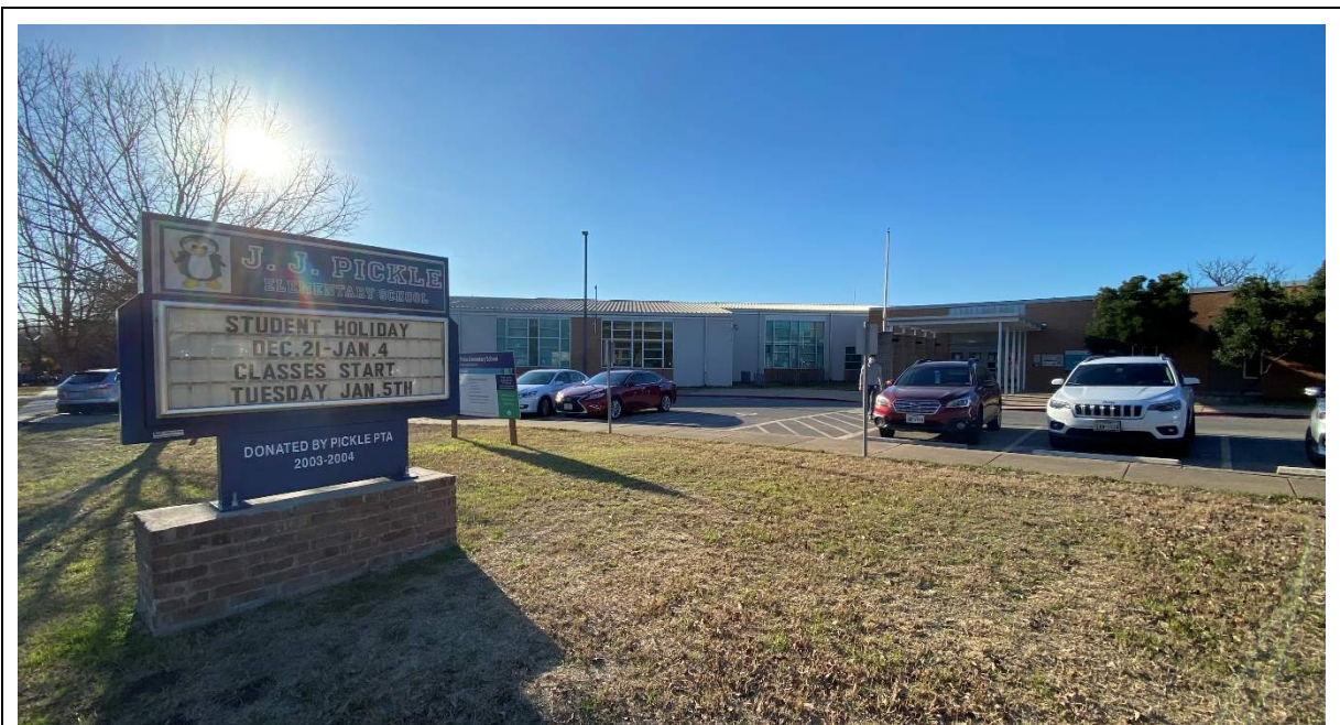
Exterior: Monument sign and building entry.
