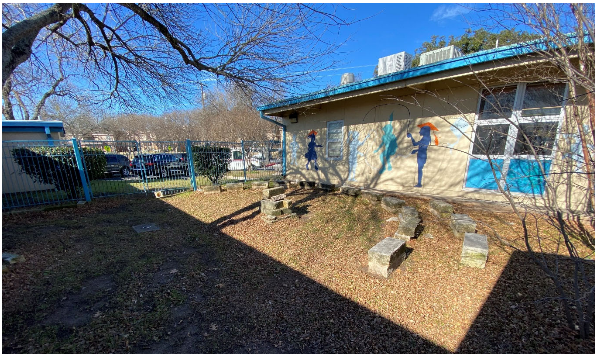
Central courtyard near the entrance serves as outdoor learning space. It needs shade and appropriate furniture to function well.
