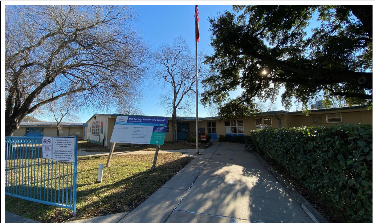
Main entrance is not clearly marked and is not directly accessible from a student drop off area.
