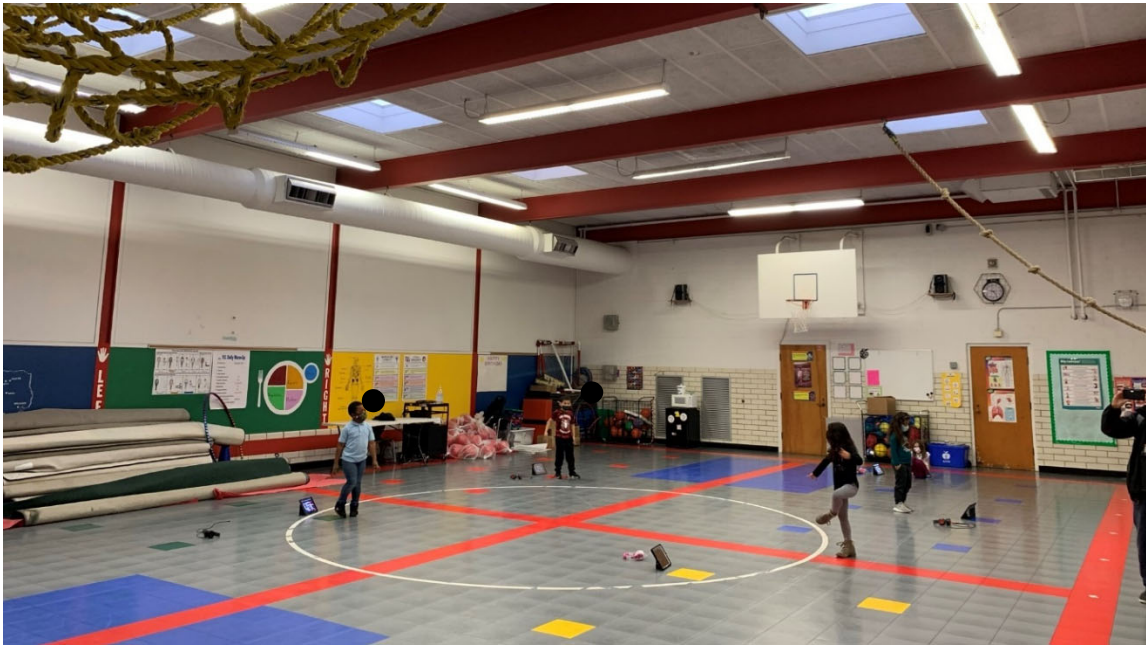
The gym is undersized and needs updates. Flooring appears to be original and there is minimal storage space.
