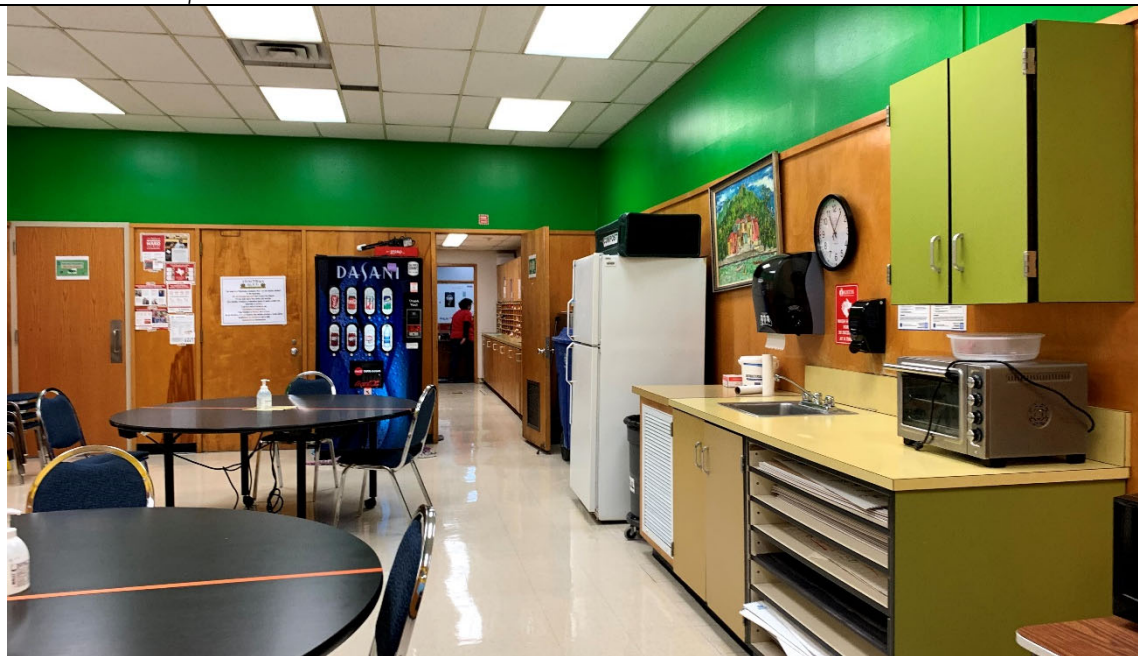
Teachers' lounge is undersized and not welcoming or seen as a place for relaxation. All administration spaces do not have access to daylight or windows.
