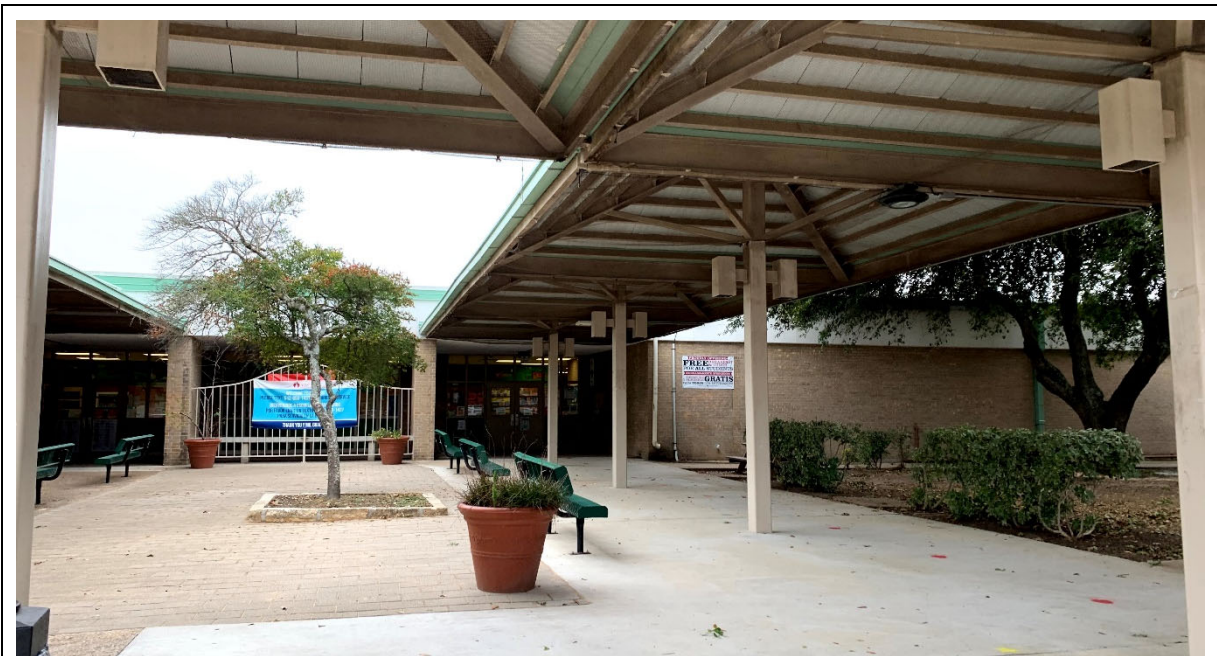
Entry Canopy: Generous canopy but limited glass at main entry.
