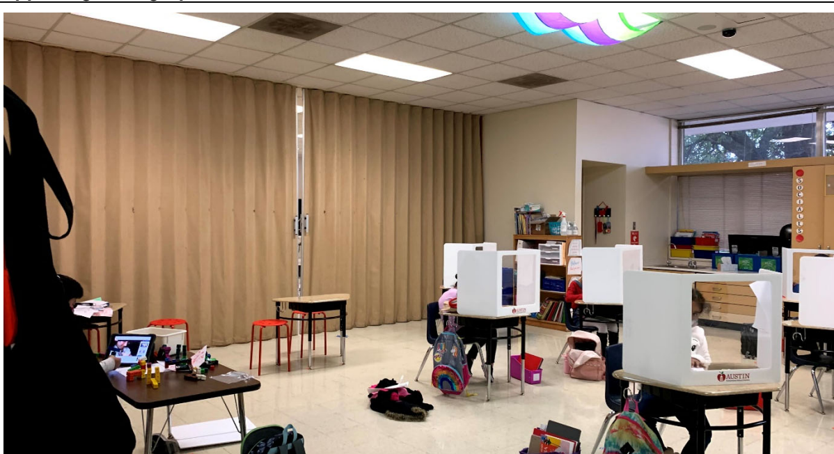
Studios (numbered 10-17) have accordion partition. They are not used very often and create acoustical issues.
