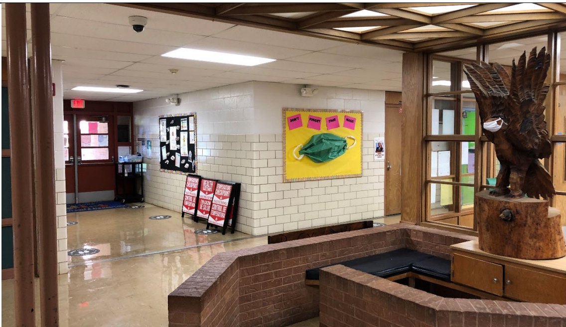
Front entry doors of building near main office. No secure vestibule on campus and allows for visitors to bypass checking in at the main office.
