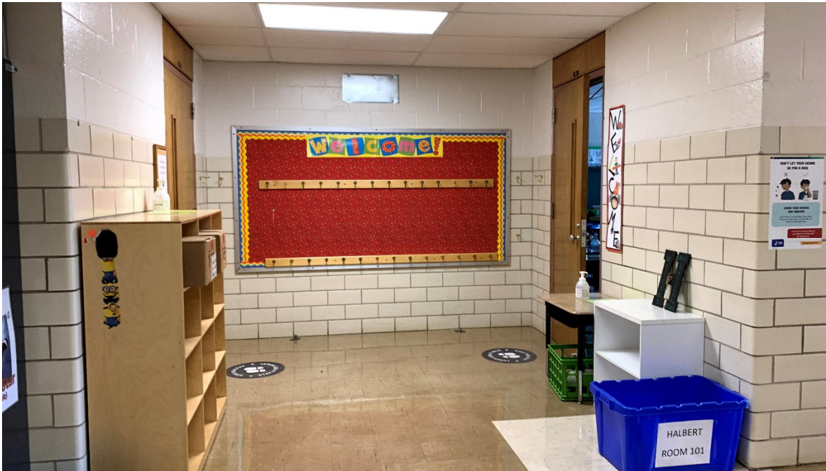
Typical entry to classrooms. Doors have minimal windows and very limited transparency for supervision in the corridor.
