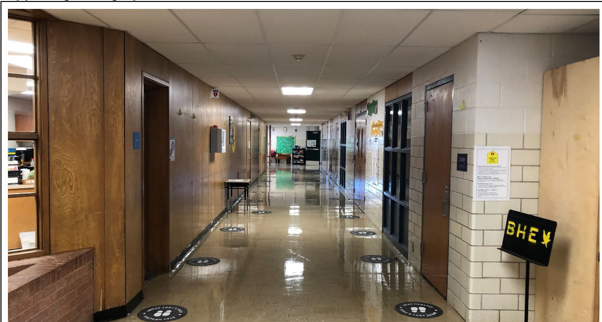
Circulation in corridors wide to allow safe and effective passage for students. Low ceiling and lighting makes the space feel unwelcoming.
