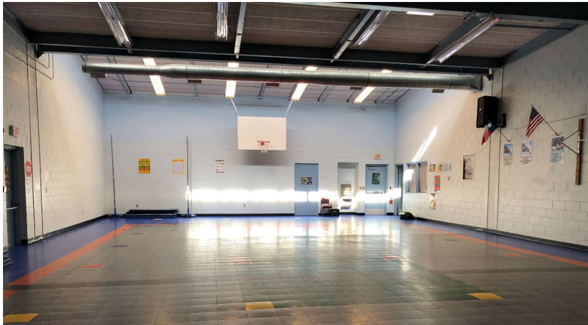
Gym is adequately sized and has some access to daylight but needs finish updates*. Storage space is inadequate and disconnected. *Gym floor was replaced after assessment walk in December 2020.
