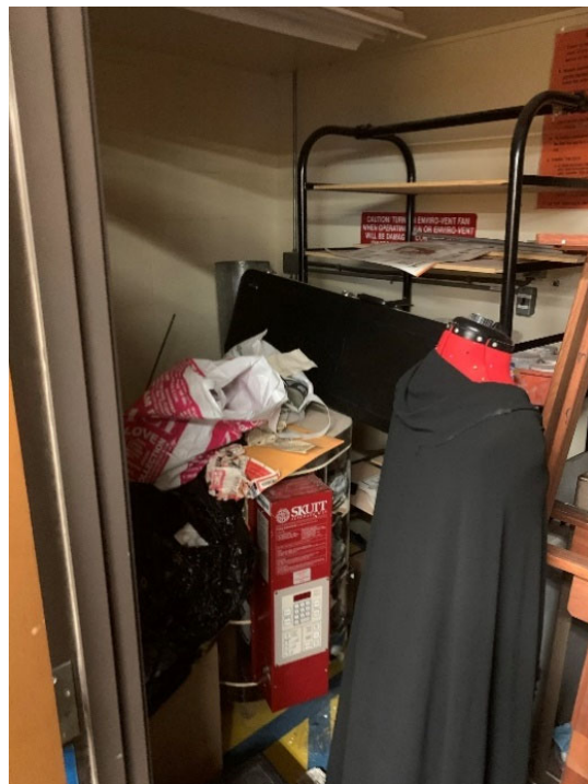
Broken kiln now serving as space for additional storage. More storage and power needed.
