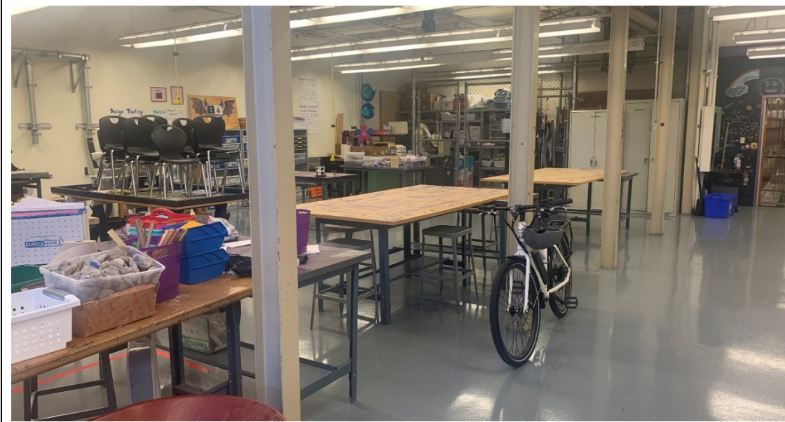
Maker space/wood shop (Room 112) is in good shape and well used. Adjoining classroom with additional technologies (3D printer) is available. During large rain events, the room does flood where an overhead coiling door used to be located. Floor has recently been replaced and a dust collector was added. The HVAC in this room will be replaced in summer 2022.
