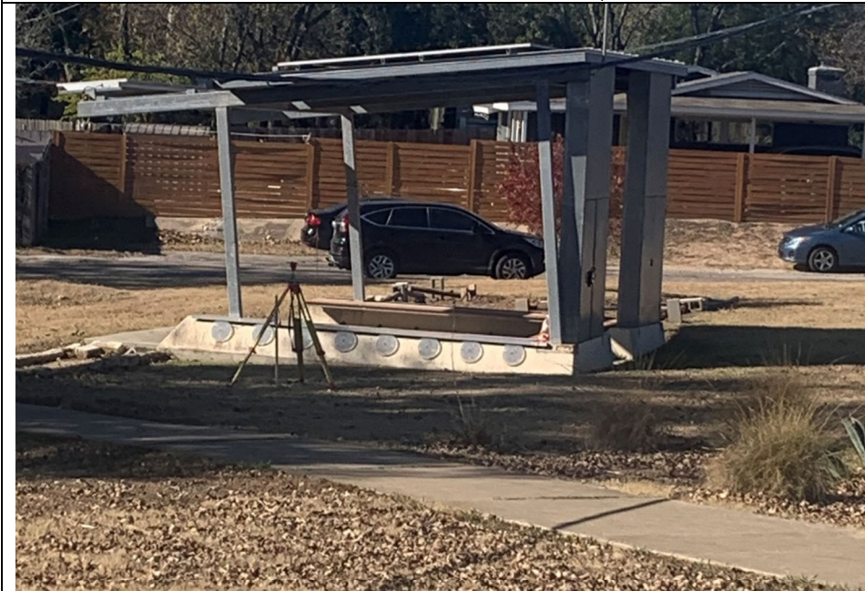
Outdoor studio space: Pavilion for outdoor learning but is far removed from school building and not flexible in its use.
