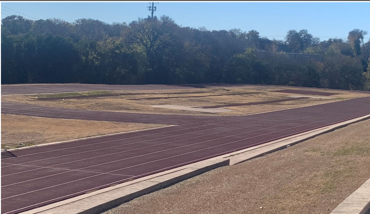
Track is undersized at 1/8 th mile and steep grade from the school to the track is problematic.
