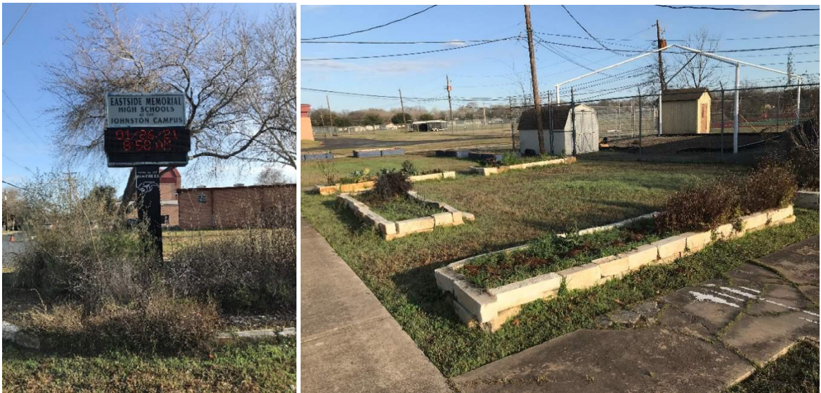
The marquee sign is far from the main entry and is overgrown with weeds (left). School gardens are present, but the unraised beds and cracked walkways are not ADA compliant (right).
