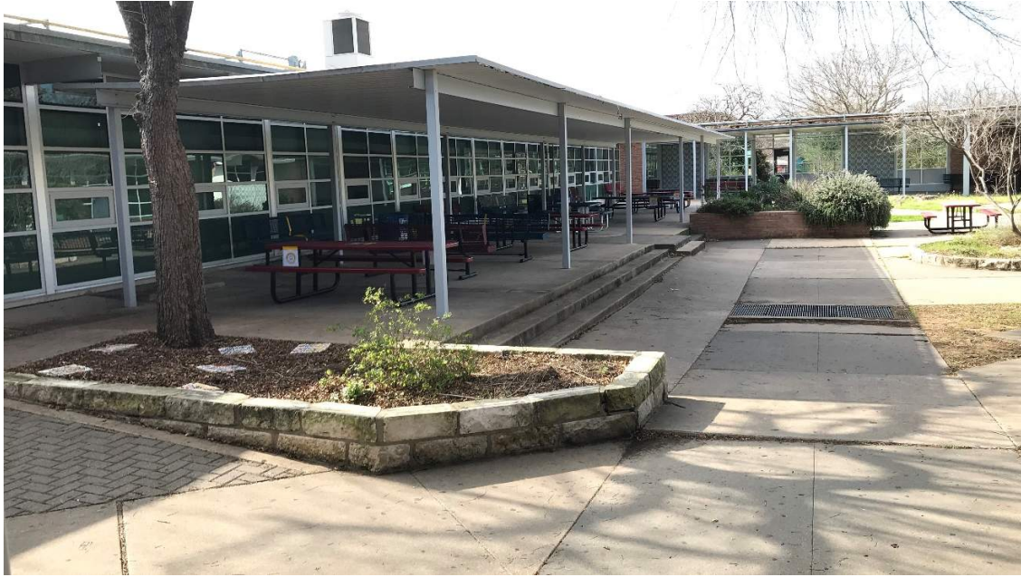
The campus has plenty of courtyards that bring in natural light and provide opportunities for outdoor learning and dining. Renovations are needed to bring some of the courtyards into ADA compliance.
