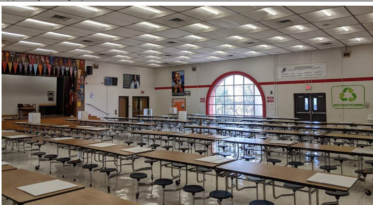
Cafeteria is undersized but in generally good condition.
