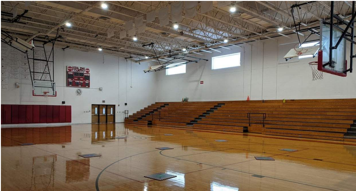
Gym bleachers are stuck in the out position, limiting flexibility of space.
