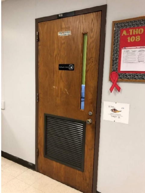
[redacted] and the louvers cause sound to travel from studios into the corridors.
