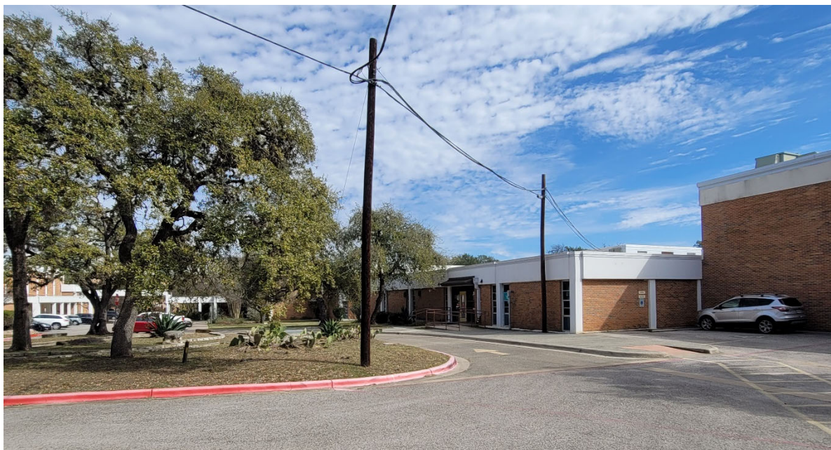
Brick and painted concrete are in good condition and feel solid.
