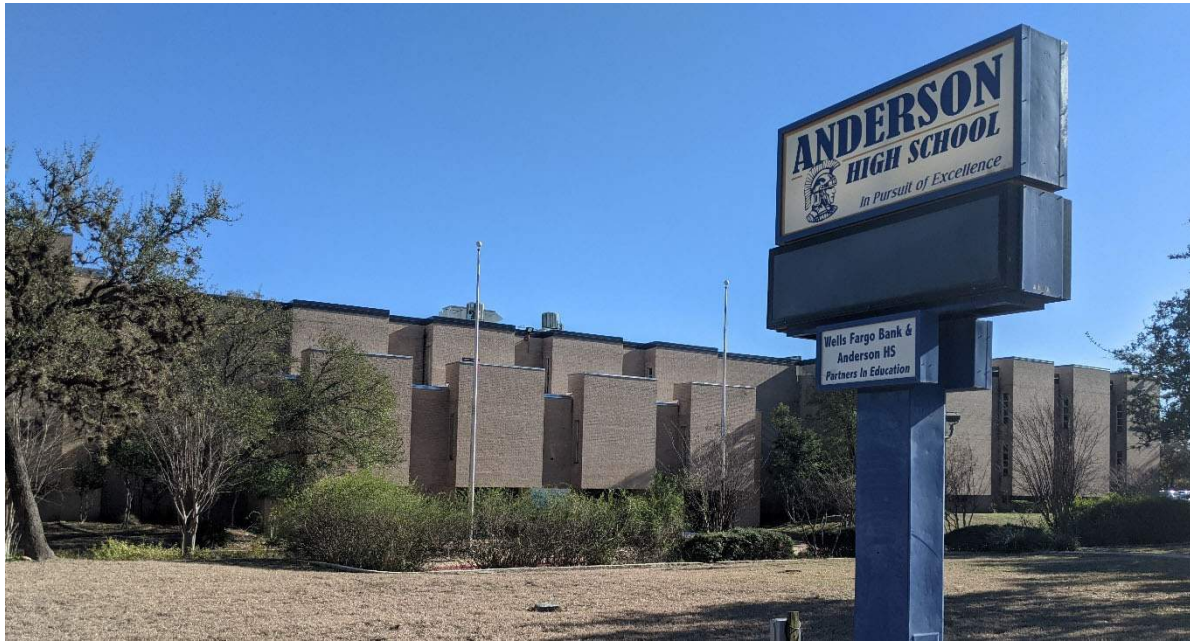
Monument sign at main drop-off. No entry canopy or building signage.
