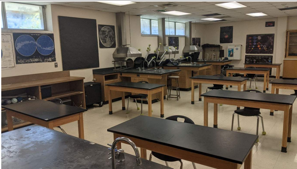
Academics & Learning: Science lab with small clerestory windows. Furniture is dated but in adequate condition. It was noted by the District Project Manager that in many locations the casework is in poor condition and should be replaced.
