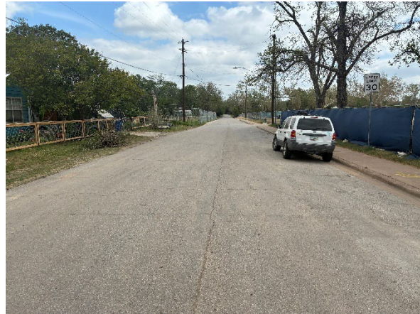
Mansell Ave Frontage Facing North
