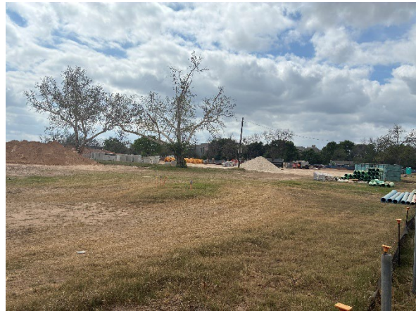
Typical View of Subject
