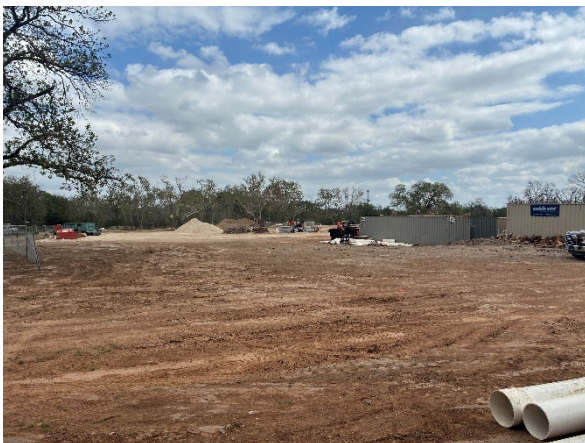
Typical View of Subject
