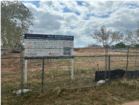
Typical View of Subject
