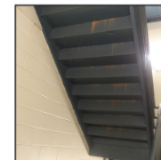
Interior Stairs Corroded Underneath
