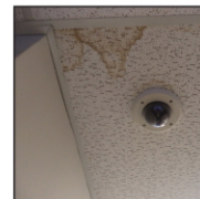
Interior Ceiling Finishes Damaged & Stained Tile
