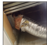
Mechanical / HVAC Damaged Insulation
