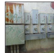
Electrical Distribution Corroded & Out of Date
