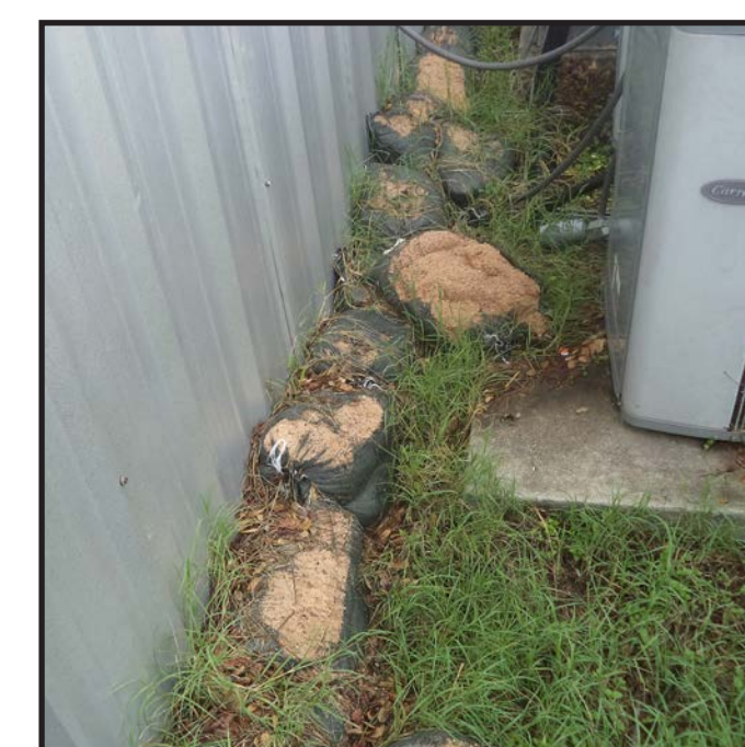
Exterior Walls Water Leakage; Ineffective Sandbags
