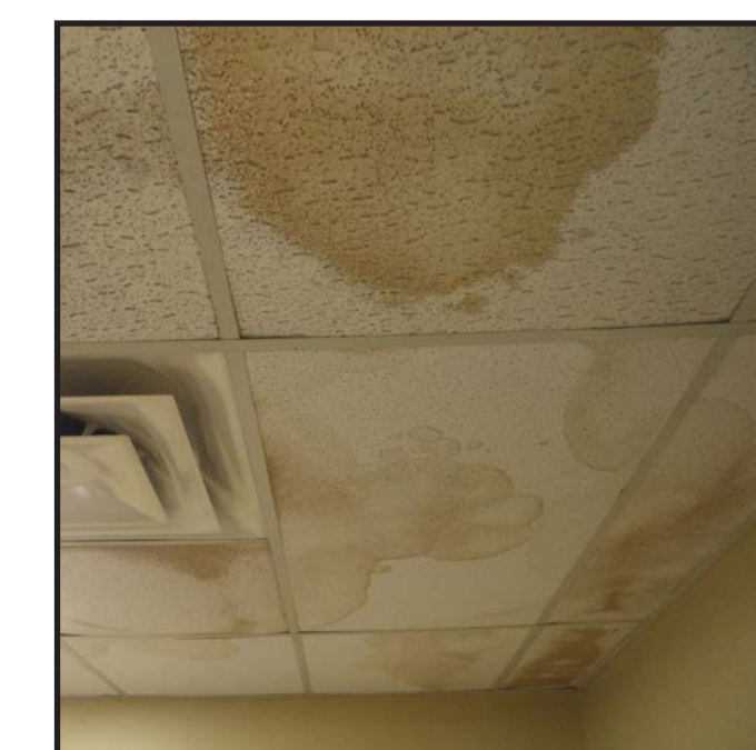
Interior Ceiling Finishes Ceiling Tiles with Water Damage
