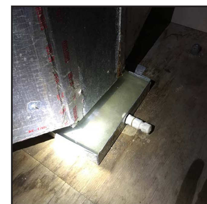
Mechanical / HVAC Drip Pans Overflowing Causing Ceiling Damage
