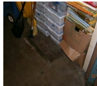
Storage on floor hatch prevents access to crawl space
