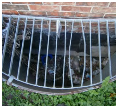
Bottom of areaway clogged with soil and debris
