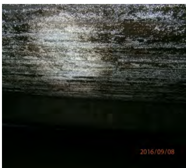
Condensation on slab underside
