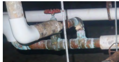
Degraded/missing pipe insulation
