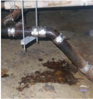
Damp soil under leaking pipes
