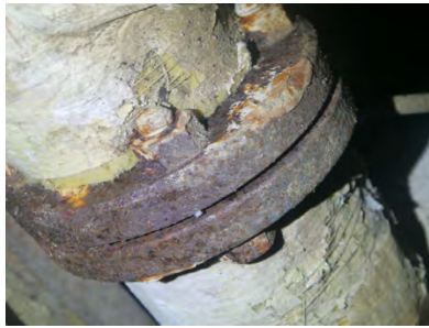
Rusted cast iron pipe connection
