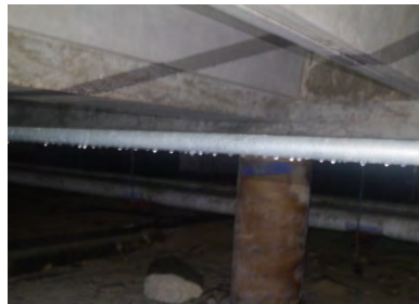
Condensation on pipes
