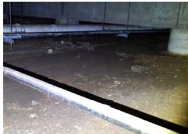
Damp soil around perimeter of building
