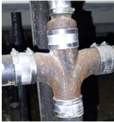
Rusted cast iron pipes
