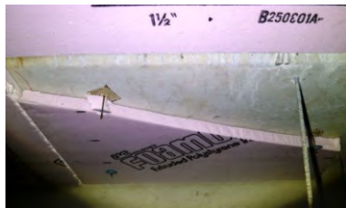
Missing rigid board insulation
