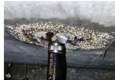
Condensation under slab
