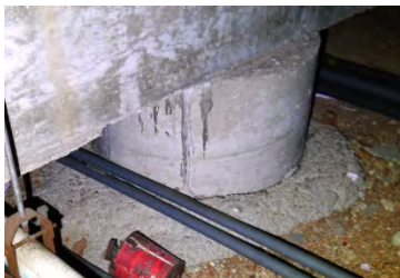
Mushrooming concrete at top of pier
