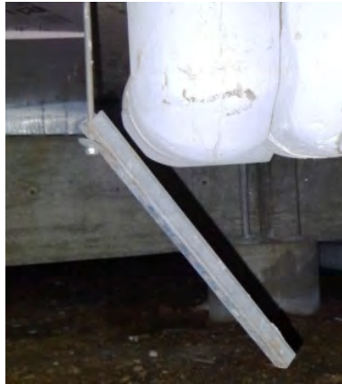
Broken pipe support
