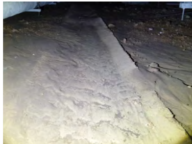
Drainage flume clogged with soil
