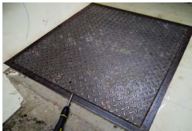
Missing floor hatch handle
