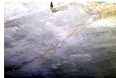
Crack in slab at corner of hatch opening
