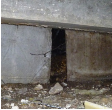
Gap between soil retainers
