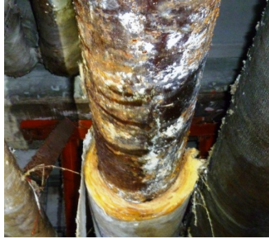
Corroded cast iron pipe
