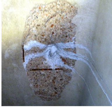
Spalling on underside precast deck
