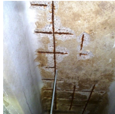
Exposed/corroded reinforcement at precast deck soffit
