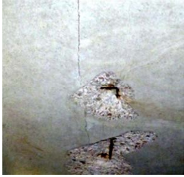
Longitudinal crack, spalling, rusting rebar in precast deck soffit
