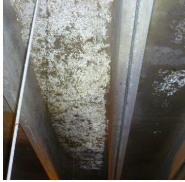
Condensation under slab
