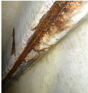
Severe longitudinal spalling and rebar corrosion at bottom of precast joists
