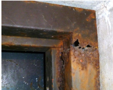
Corroded access hatch frame
