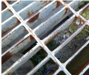
Mild corrosion on areaway grate
