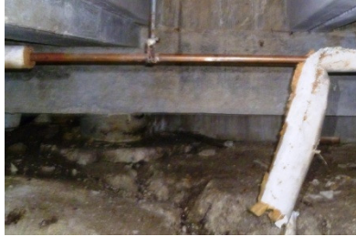
Fallen/degraded pipe insulation
