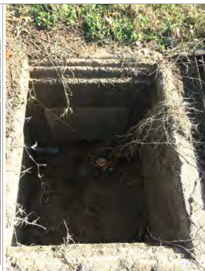
Inlet missing cover (track)
