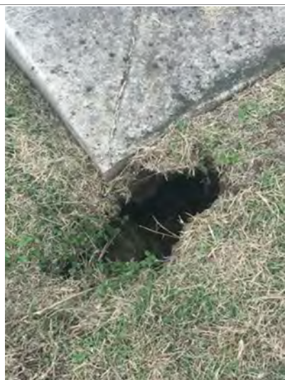
Erosion/hole around inlet
