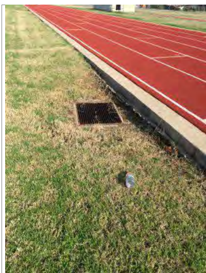
Drop off to inlet from track
