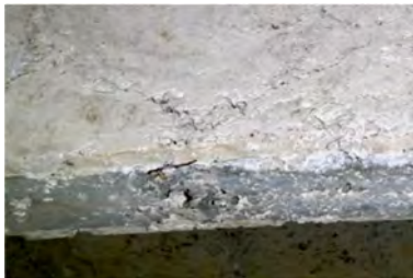
Honeycombing at bottom of pan joist
