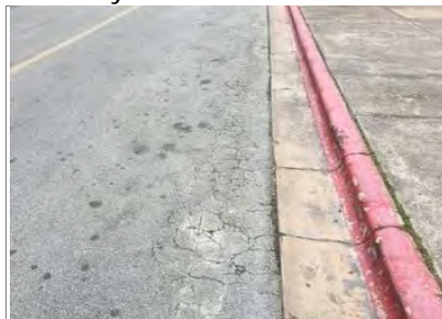
Cracking along gutter (front drop off)
