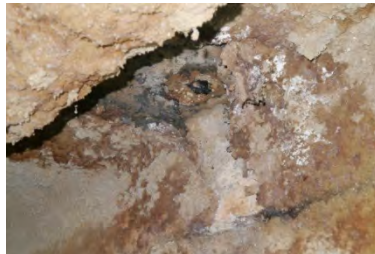
Rusted metal concealed behind fireproofing
