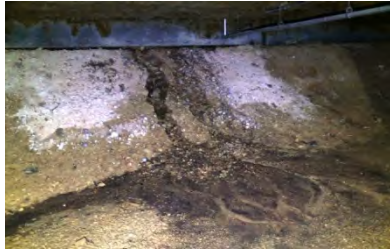
Water infiltration at perimeter
