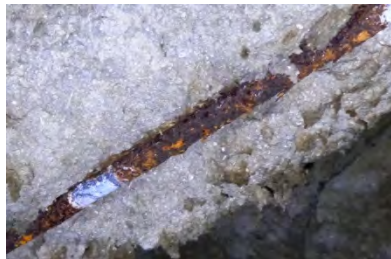
Rusted pipe under joist
