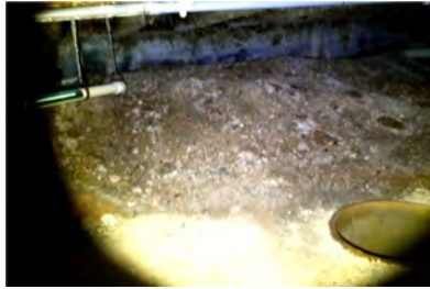
Damp soil at perimeter
