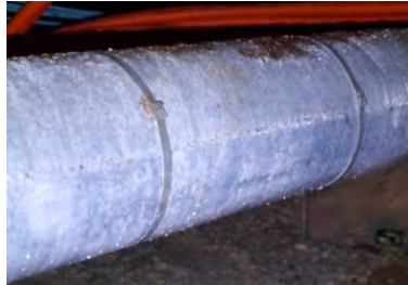
Condensation on pipe
