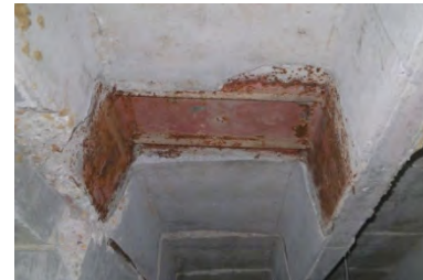
Metal pan form left in place and corroding
