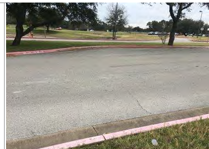
Block cracking (front entrance drive)
