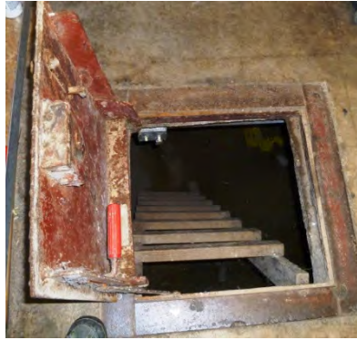
Rusted access hatch
