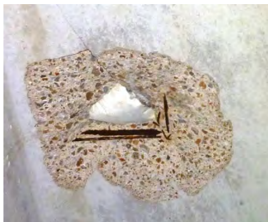
Deck spall and exposed/rusted slab reinforcement
