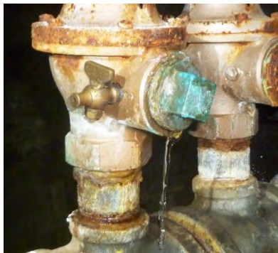
Badly leaking pipe
