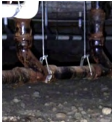
Rusted cast iron pipes
