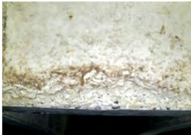
Honeycombing in pan joist diaphragm
