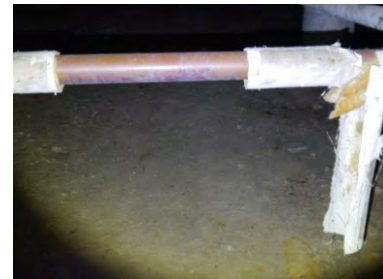
Missing/degraded pipe insulation
