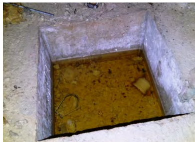
Standing water in drainage pit
