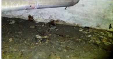
Saturated soil at perimeter
