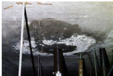
Condensation under slab
