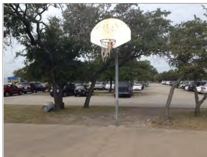
Deteriorated rim and backboard
