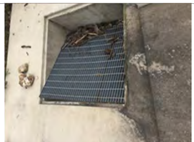
Outfall grate collapsed
