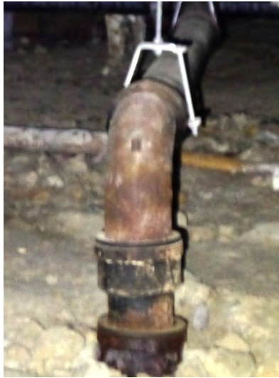
Slightly rusted Pipe
