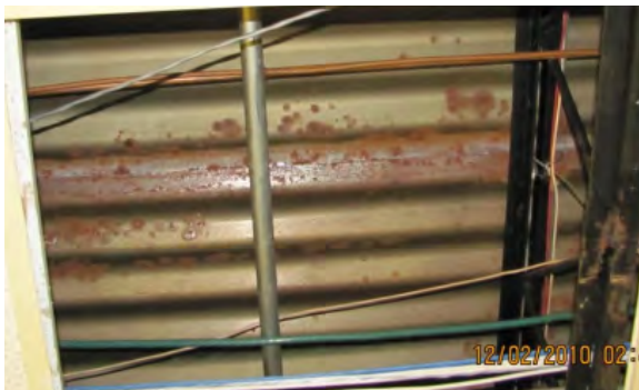
Advanced roof deck corrosion
