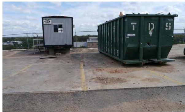
300 Wing floor framing is currently being used to support a dumpster and construction offices
