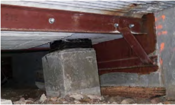
200 Wing floor framing retrofit appears in good condition
