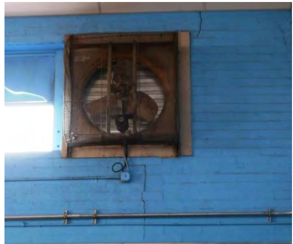
Vertical cracks on west wall
