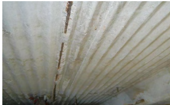
Spalling concrete deck and exposed/corroded rebar
