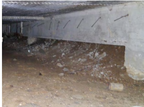
Void space below perimeter beam is filled with soil
