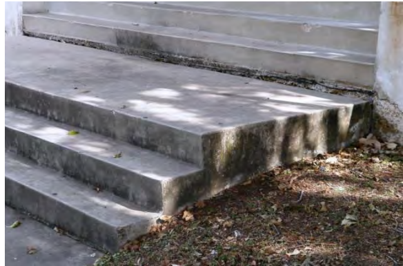
Grade-supported stairs have displaced vertically
