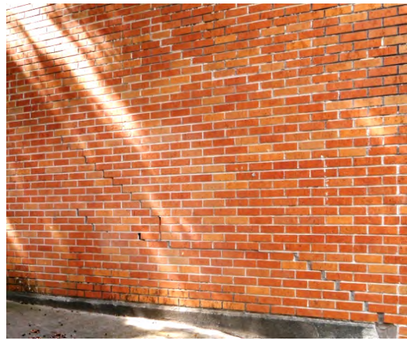
Gym recreational room diagonal cracks (some previously repaired)
