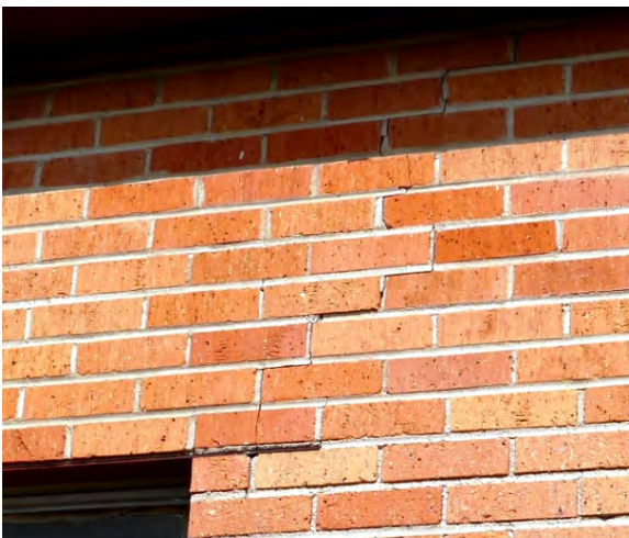
Crack at window opening on west wall of gym
