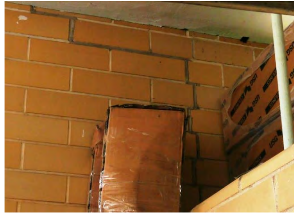
Reopened crack in Men's Locker Room
