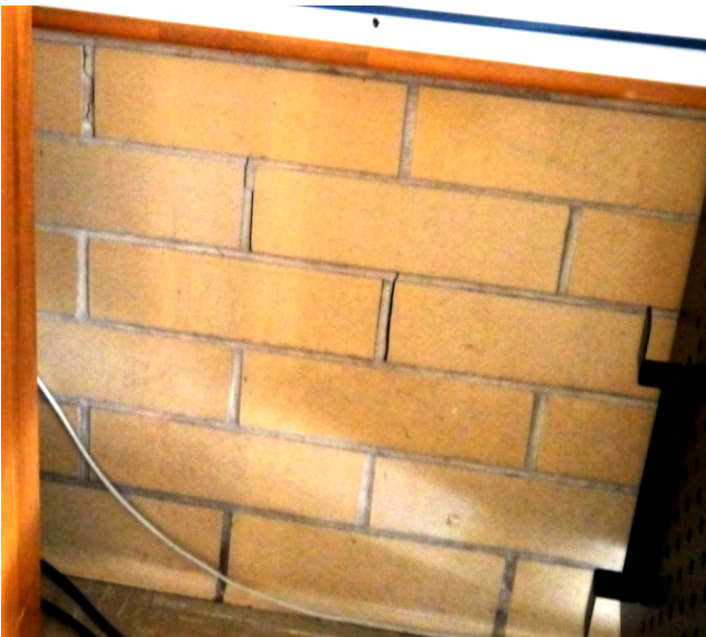
Cracks in classroom brick wall
