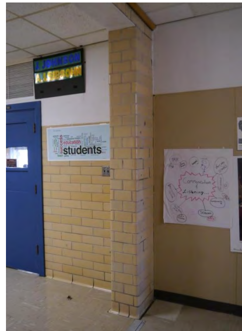
Cracks on hallway column at expansion joint between original building & 1958 west addition
