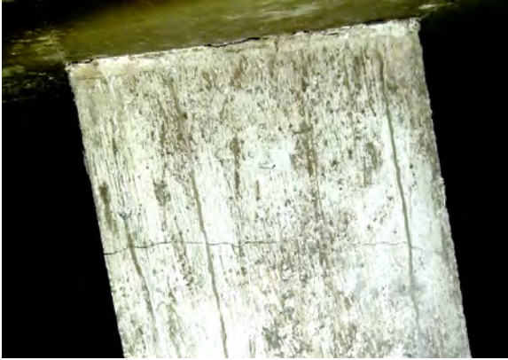
400 Wing Column Horizontal Crack
