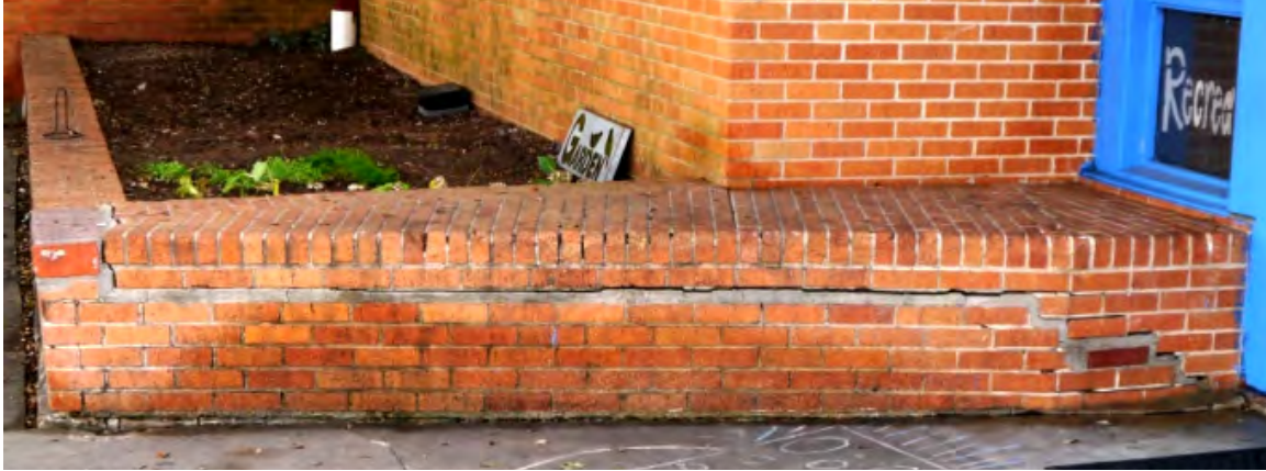
Horizontal crack on planter masonry
