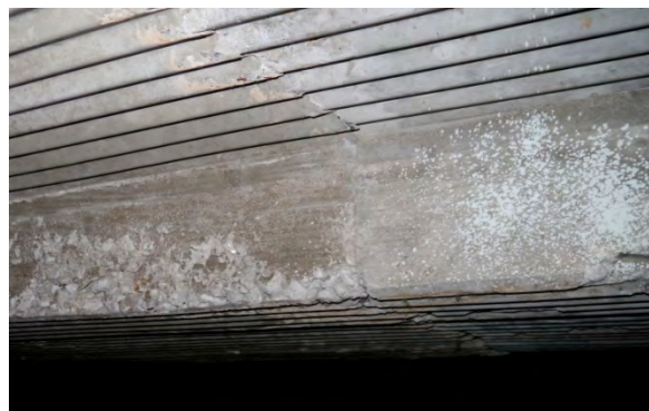
Concrete honeycombing on face of interior floor beam
