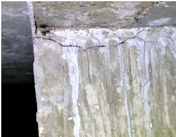
400 Wing Column Horizontal Crack
