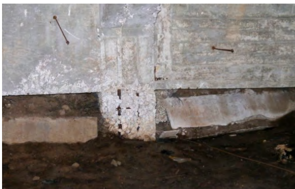
Damp soil, Failing soil retainers, Honeycombing and exposed/corroded column reinforcement
