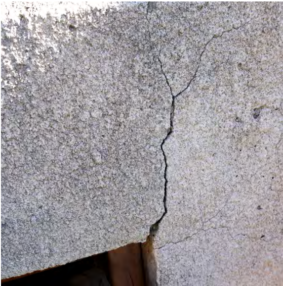
Diagonal crack at top of access hatch
