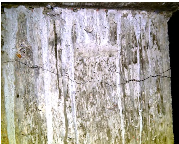
400 Wing Column Horizontal Crack
