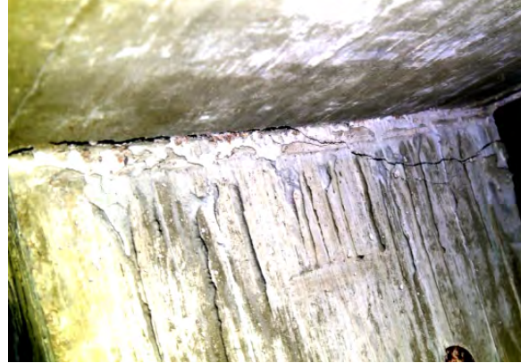
400 Wing Column Horizontal Crack
