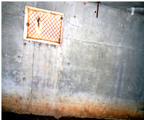
Diagonal cracks around vent opening
