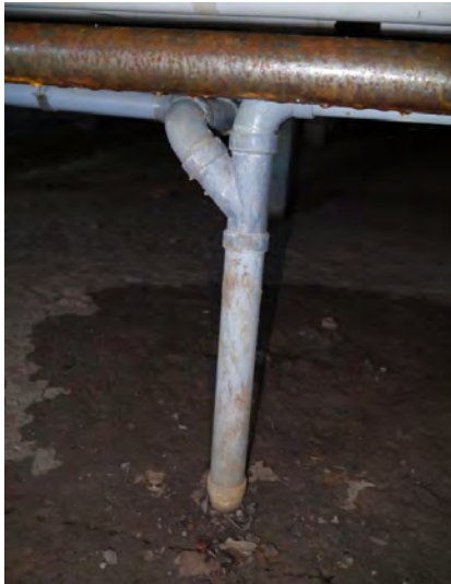
Condensation on pipes, potential pipe leak
