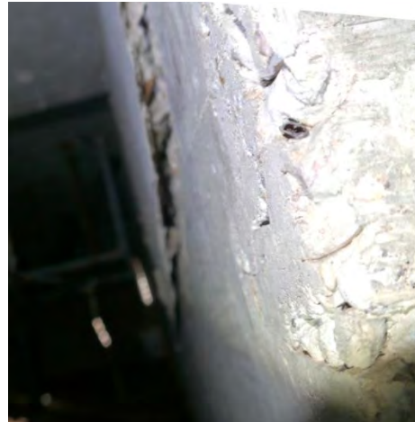
East perimeter beam is shifting eastward and pulling away from perpendicular interior beams
