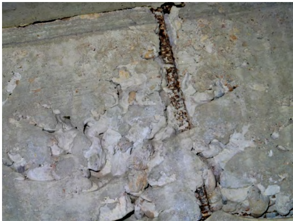
Concrete honeycombing, exposed/corroded reinforcement
