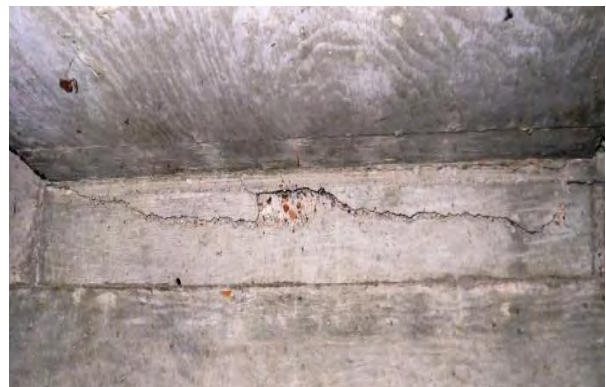
Horizontal crack under interior beam
