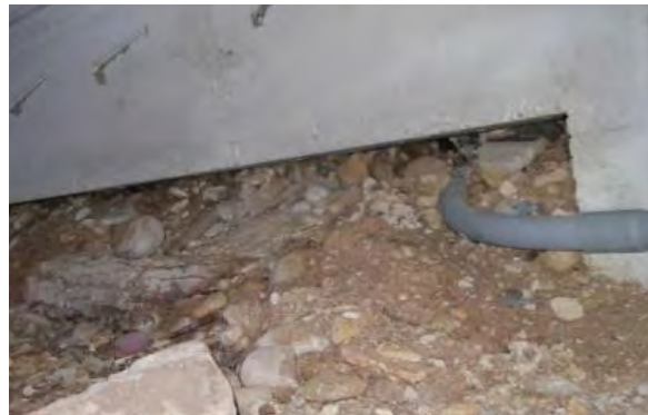
Void space below perimeter beam is filled with soil
