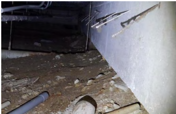
Damp soil around perimeter of building
