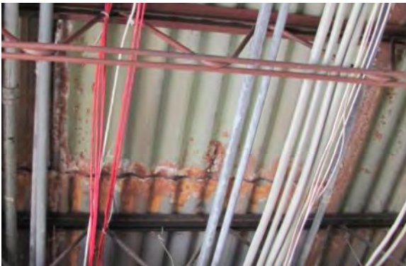
Advanced deck corrosion
