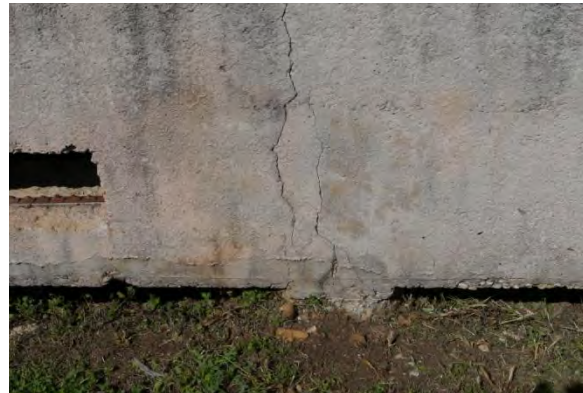
Outside face of perimeter beams show signs of structural distress
