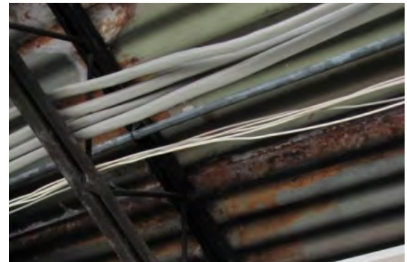
Advanced deck corrosion
