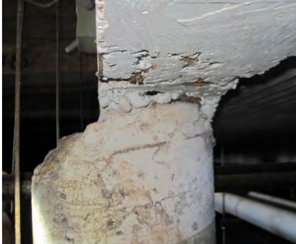
Exposed/corroded beam rebar, beam not centered over pier
