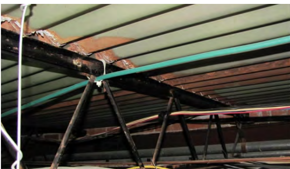
Advanced deck corrosion, joist corrosion
