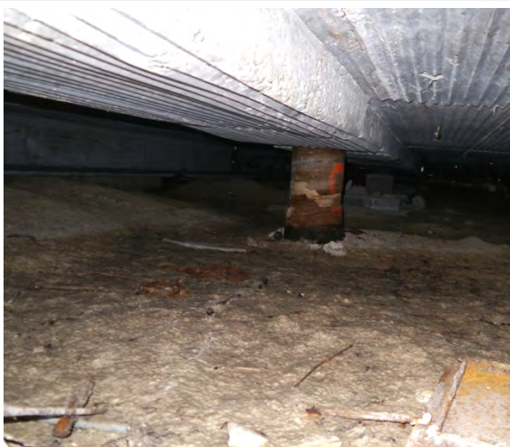
Saturated soils in crawl space
