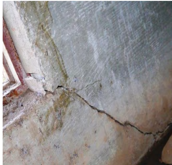
Access hatch diagonal crack from interior
