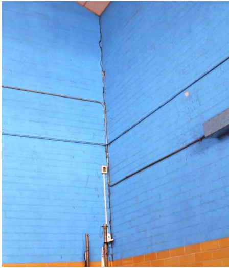
Crack on corner of main gym east and north walls
