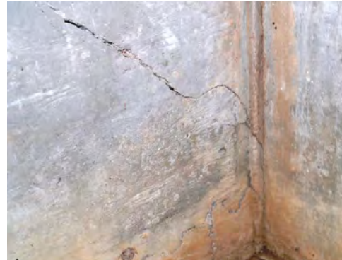
Diagonal crack at southeast corner
