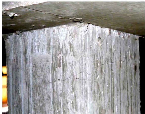
400 Wing Column Horizontal Crack
