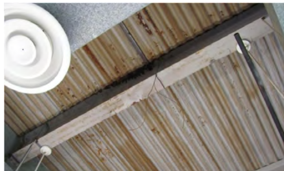
Roof deck corrosion
