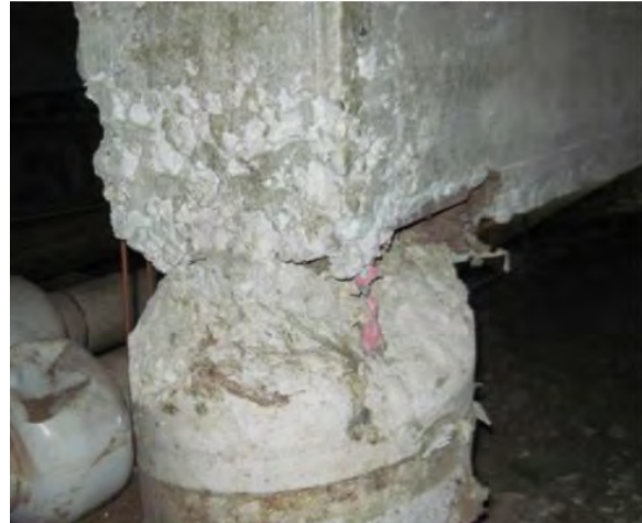
Exposed/corroded beam rebar, extensive honeycombing at pier-beam connection
