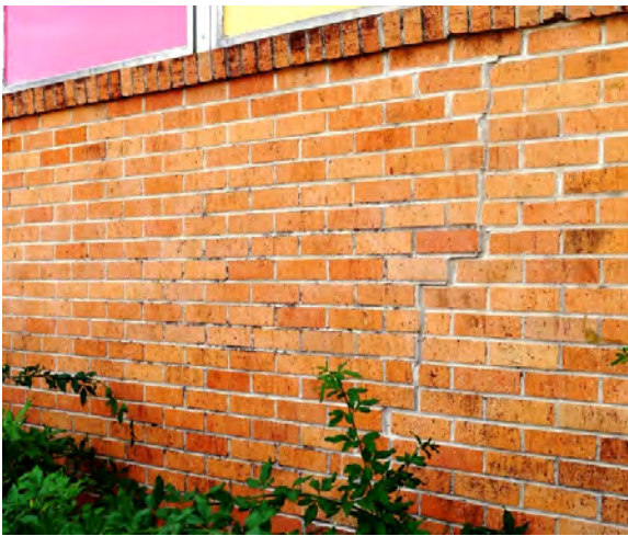
Vertical/diagonal crack below window
