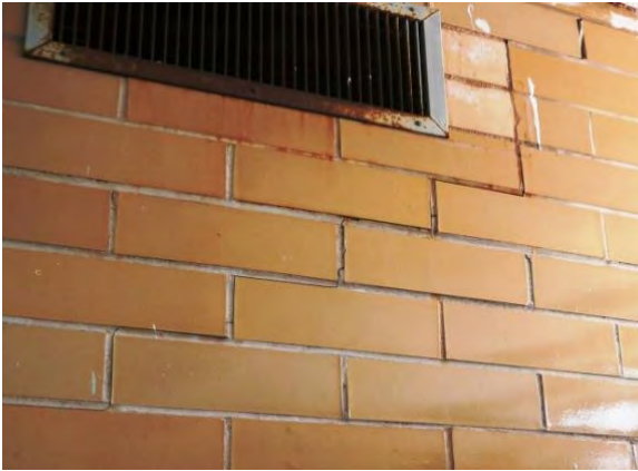
Reopened crack in Men's Locker Room
