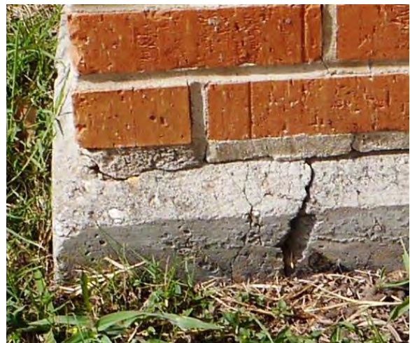
Perimeter beam crack below exterior brick
