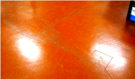
200 Wing Kitchen reopened slab cracks
