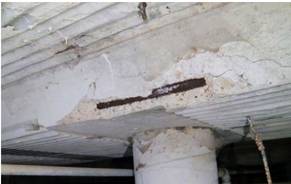
Spalling concrete interior beam and exposed/corroded rebar
