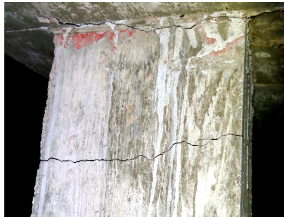
400 Wing Column Horizontal Crack
