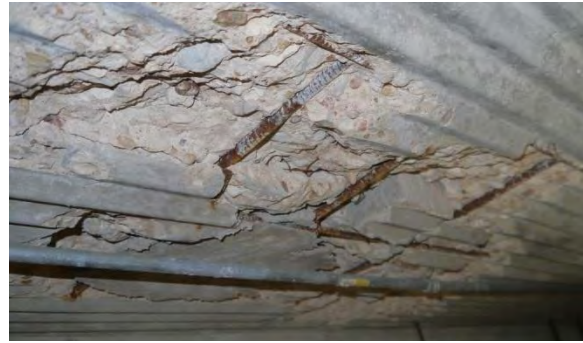
200 Wing slab spalling with exposed/corroded rebar
