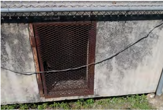
Crawl space hatch door is welded shut
