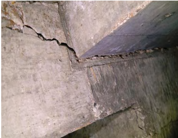
Diagonal crack on 400 Wing east perimeter beam near bottom of abutting interior beam and (near stairs)
