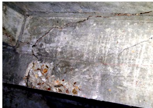
Cracks on 400 Wing east perimeter beam at abutting interior beam (near stairs)
