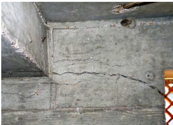
Crack from bottom of interior beam to vent
