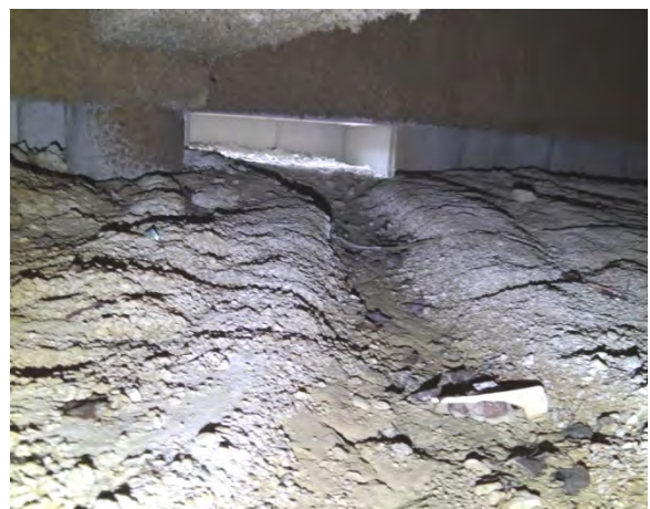
Clear Flow Lines in the Soil Leading From Areaway Openings
