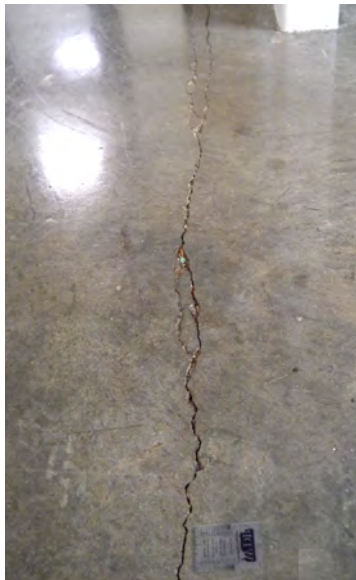
Large Slab Cracks at Corner Entryways
