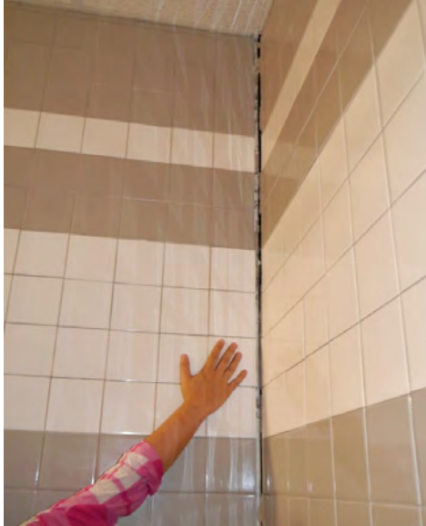
Separation at Top of Abutting Interior Walls
