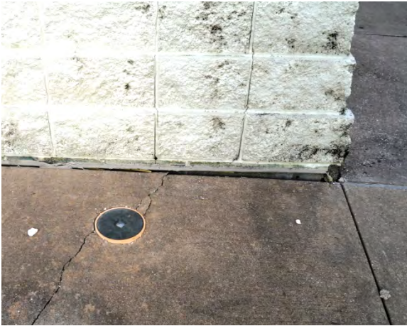
Exterior Flatwork Around Corner Column has Settled
