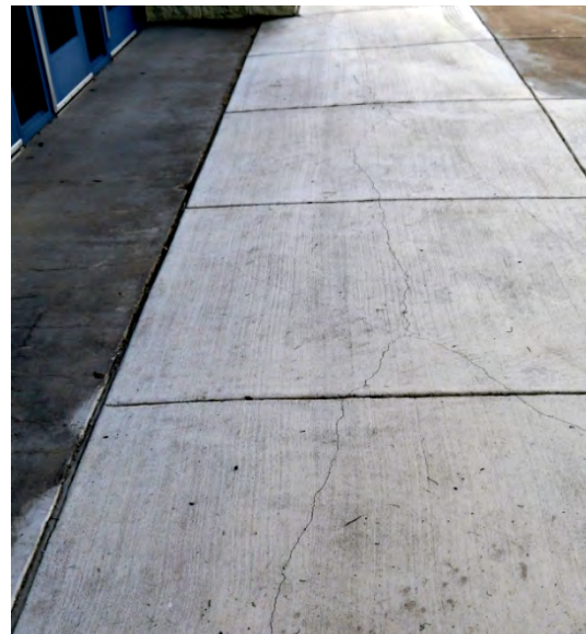
Cracks in Newly Replaced Flatwork
