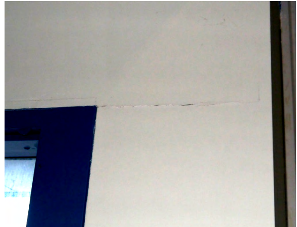
Crack in Wall Finish at Entryway Window Corner
