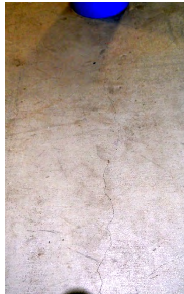
Slab Cracks at Top of Entryway Stairs
