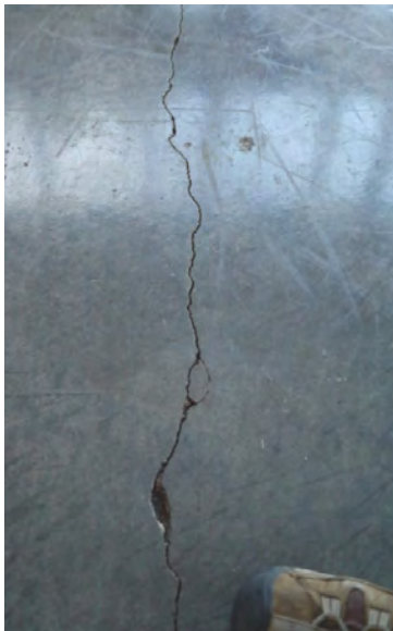
Large Slab Cracks at Corner Entryways
