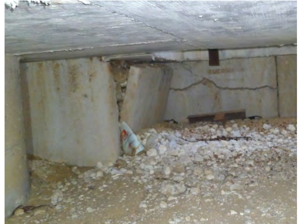
Cracked and Caving Soil Retainers
