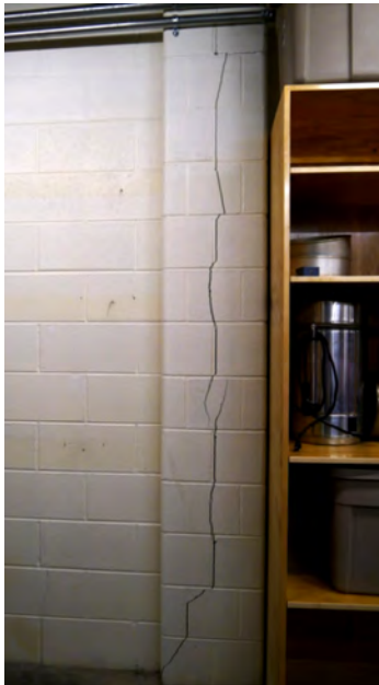
Large Vertical Crack in CMU Pilaster
