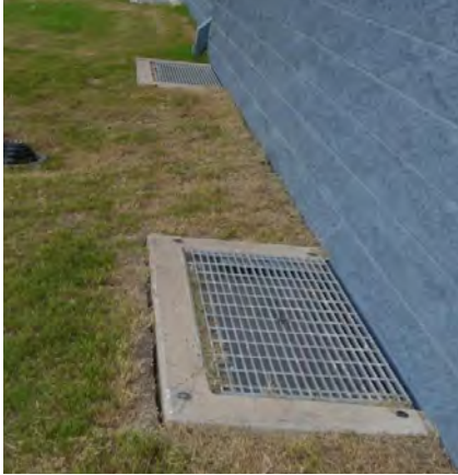
Low Areaway Curb Heights Allow Water into Crawl Space
