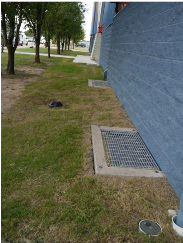
Flat Grading Around Perimeter of Building
