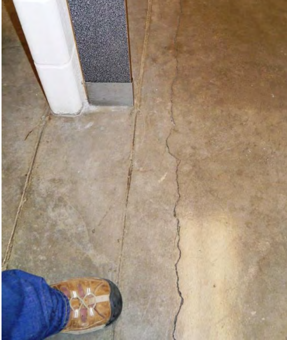
Large Slab Cracks Adjacent to Double Control Joints
