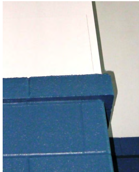
Wall Finish Damage Above CMU Pilaster in Outer Corridor
