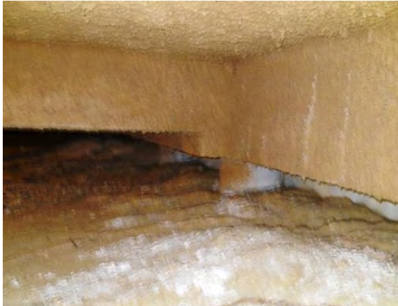
Concrete Floor Framing Obscured by Spray Fireproofing
