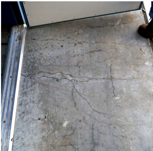
Exterior Topping Slab Cracks at Corner Entryways
