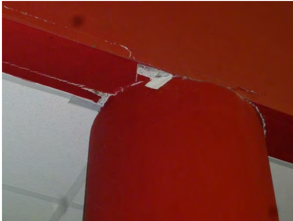
Finish Damage at Top of Red Column Near NW Entryway
