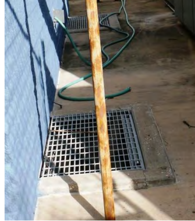
Low Areaway Curb Heights Allow Water into Crawl Space
