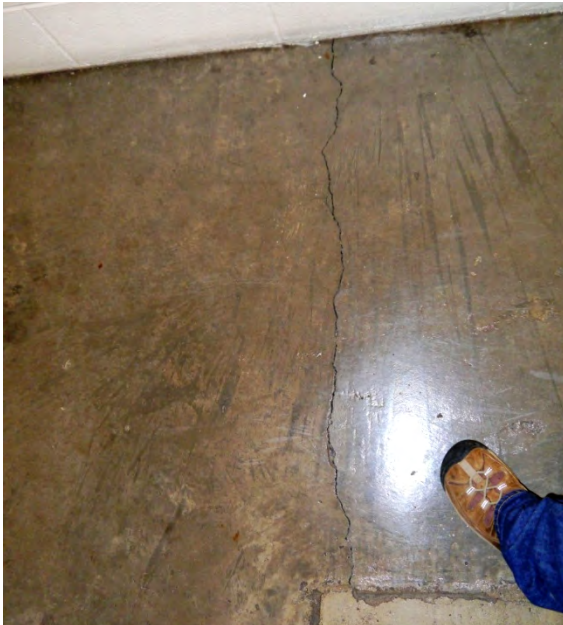
Slab Topping Crack in Walkway in Front of Bleacher Seating
