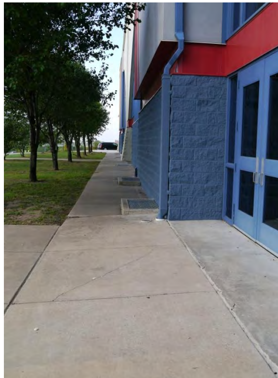
Flat Grading Around Perimeter of Building
