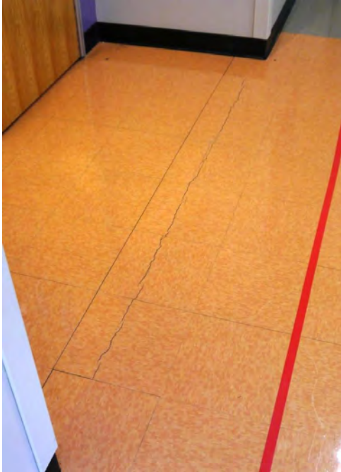
Cracked floor tiles near west library door
