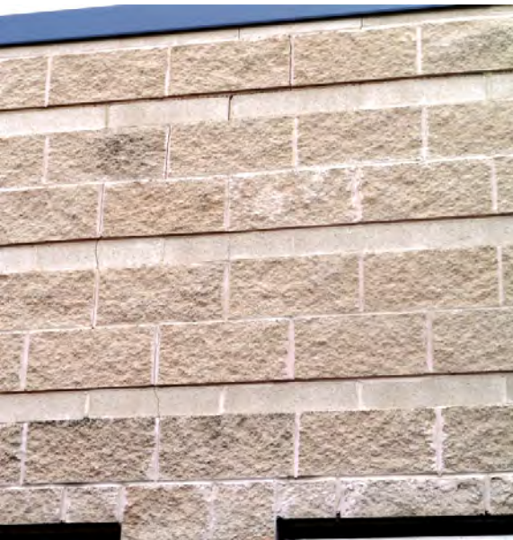
Crack over window
