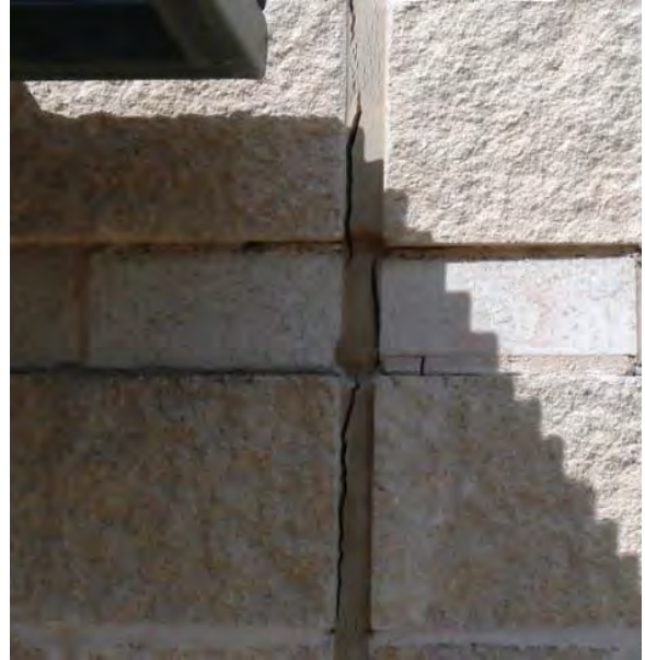
Separation at expansion joint
