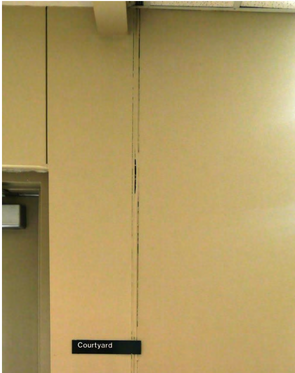
Separation at expansion joint
