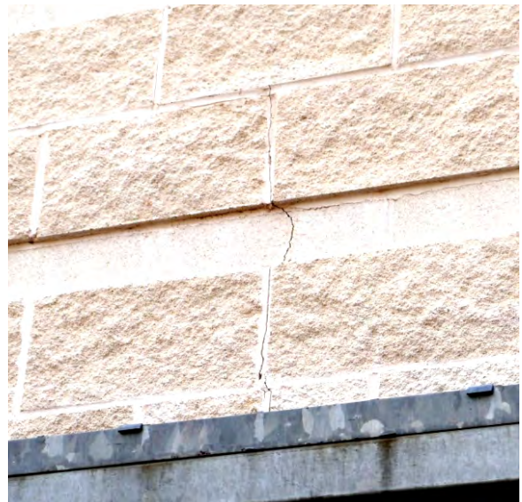
Crack over window
