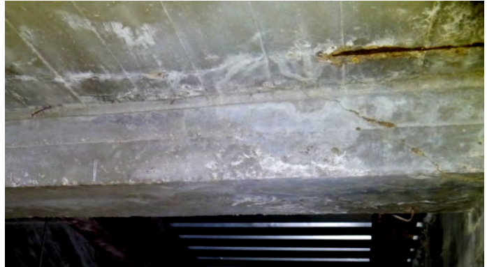
E-W Crack in Bottom of Slab Parallel to Beam
