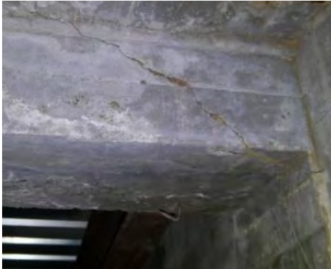
Diagonal Crack in Beam at Top of Stair
