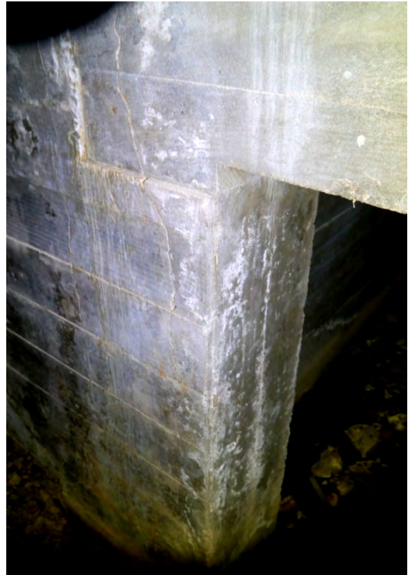
Vertical Cracking in East Wall
