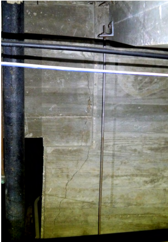
Vertical Cracking in West Wall
