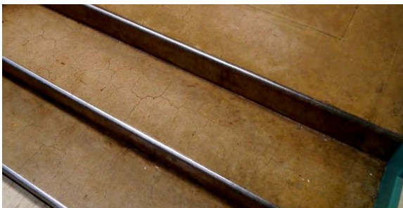
Shrinkage Cracking in Stairs
