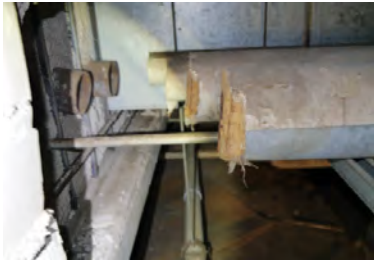
Abandoned and cut pipes
