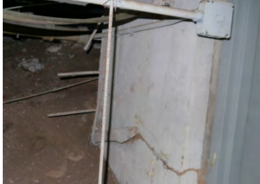
Exposed rebar from previous demolition and repaired crack in wall
