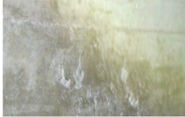
Minor spalling and honeycombing in wall
