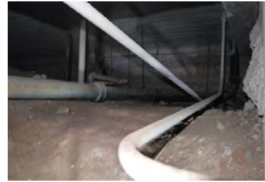
Pipes bearing on soil
