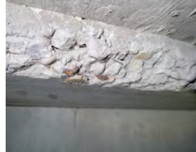
Minor spalling at corners of beams
