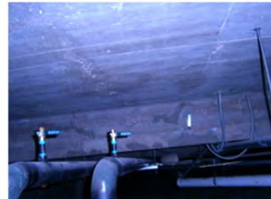
Minor spalls under slab at Access Point 3
