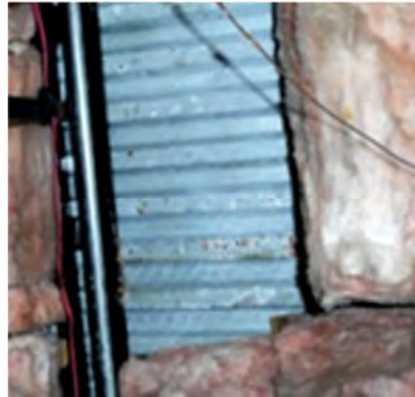
Minor rust on underside of metal floor deck
