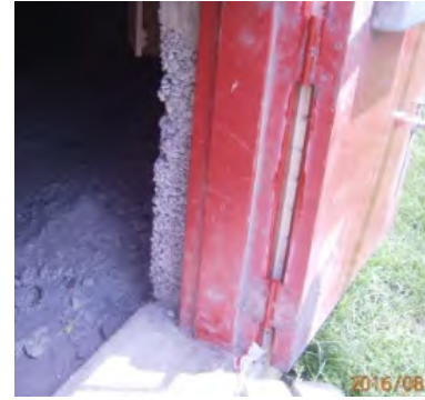
Honeycombing at perimeter wall at access door
