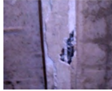
Exposed and rusted reinforcement in webs of pan form slab near Boiler Room
