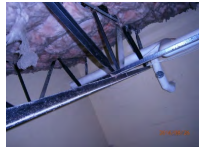
Batt insulation deteriorating
