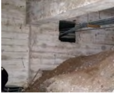
Some cracking around holes cut in perimeter walls, patching near boiler room
