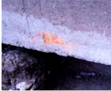
Minor honeycombing on perimeter beam
