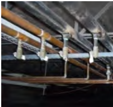
Rust on pipes
