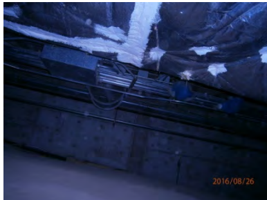
Damage to and patching of duct insulation
