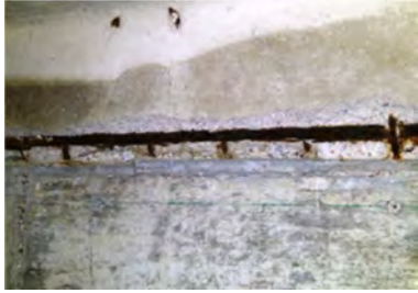
Exposed reinforcement in precast joist
