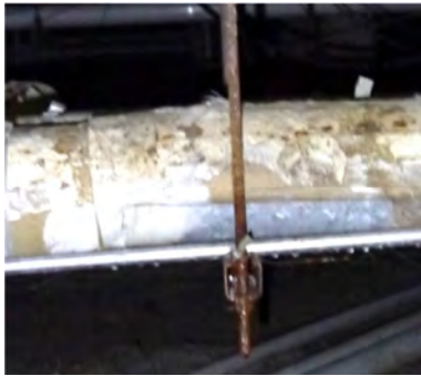
Rusted pipe hangers, degraded pipe insulation
