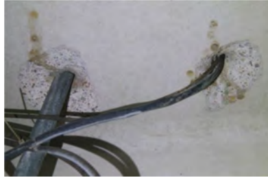
Spalling under deck
