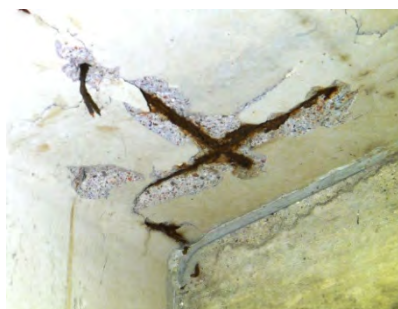
Exposed reinforcing underside of slab
