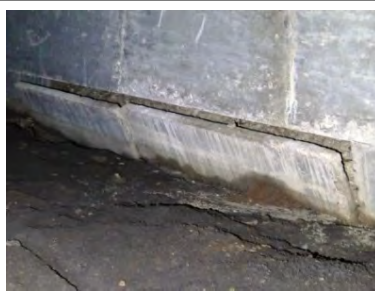
Overturned concrete soil retainers
