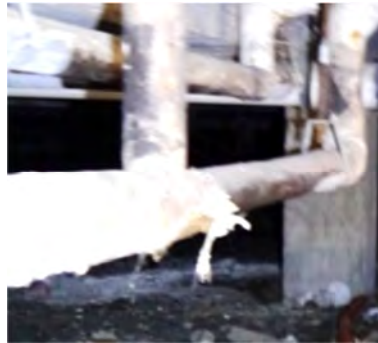
Stripped pipe insulation
