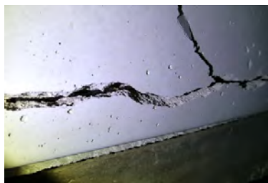
Longitudinal cracking in precast joist
