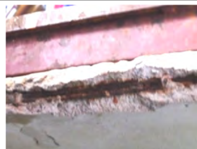
Exposed slab reinforcement below hatch
