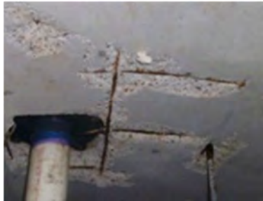
Spalling & exposed/corroded reinforcement at underside of precast pan joist flange
