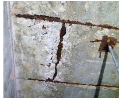
Exposed/corroded reinforcement in bottom of slab due to insufficient clear cover
