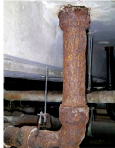
Rusted cast iron pipe
