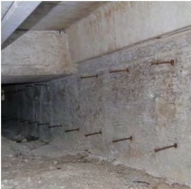
Corroded form ties at perimeter beams
