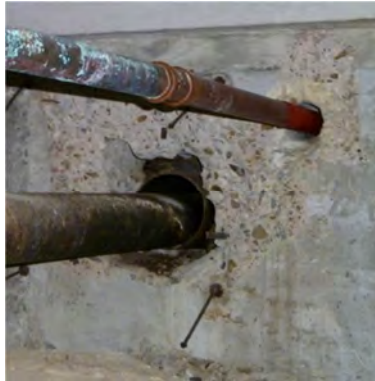
Honeycombing/spalling in perimeter beam at pipe penetration
