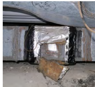
Degraded duct insulation
