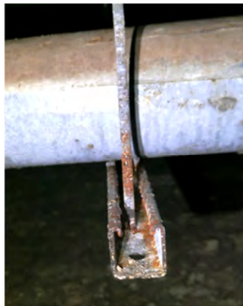
Corroded pipe hangers
