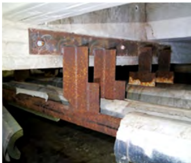
Corroded pipe supports
