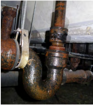
Wet/leaking pipe, corrosion
