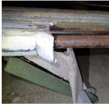
Failed pipe insulation
