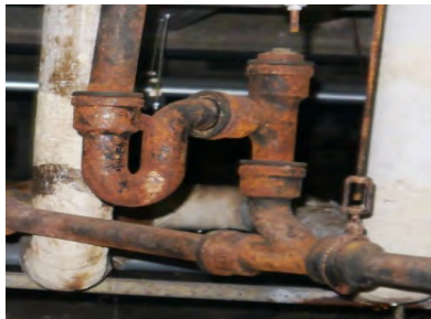
Rusted pipes & pipe supports
