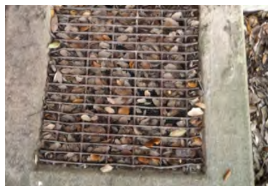
Foliage partially clogging areaway
