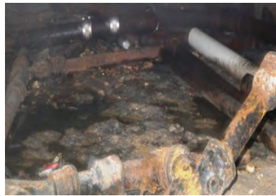
Water under kitchen pipe leak
