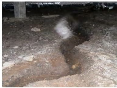
Damp soil, water intrusion from building perimeter
