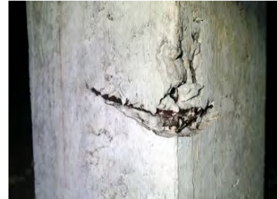
Spalling at column corner, Exposed/corroded column reinforcement
