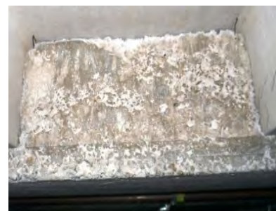
Honeycombing on interior beam
