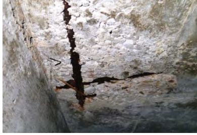
Exposed/corroded rebar and honeycombing under flat slab
