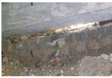
Failed soil retainers
