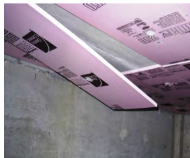
Falling rigid board insulation
