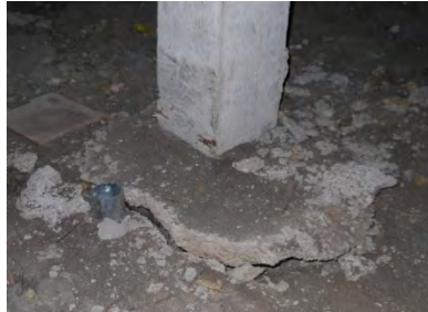
Concrete mushroom at top of pier
