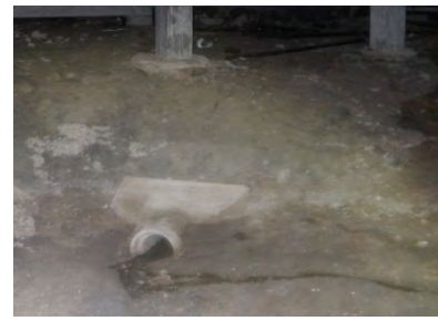
Partially clogged drain
