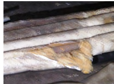
Torn/degraded pipe insulation
