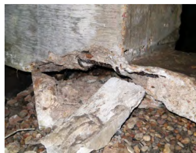
Large spall under former perimeter beam (adjacent to library addition)
