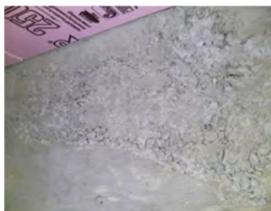
Honeycombing on face of perimeter beam
