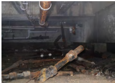
Pipe leak in slab, broken pipe, and broken pipe hanger. Mistiness of picture is due to steam in the air.
