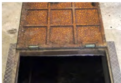
Corroded floor access hatch frame & door
