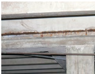
Exposed/corroded longitudinal rebar at bottom of precast channel leg
