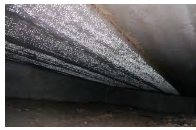
Poor ventilation, Condensation under slab
