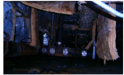
Saturated and collapsing insulation
