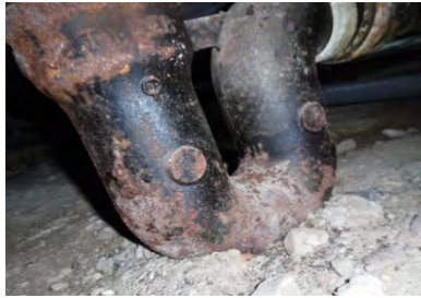
Pipe bend touching soil and rusting
