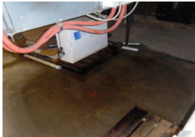
Pool of water under HVAC
