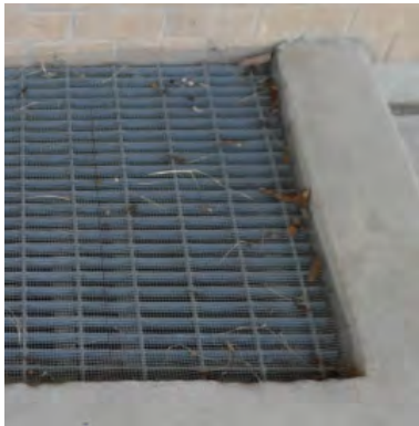
Areaway welded shut
