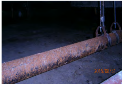
Rusting on pipe and pipe hangers
