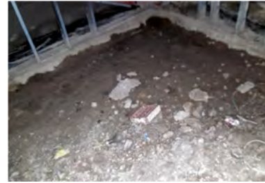
Damp soil around perimeter of northwest crawl space
