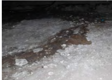
Water infiltration from under east perimeter
