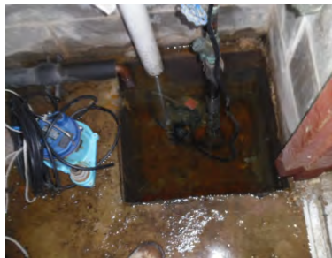
Pit holding water outside northwest access to crawl space, sump turned off
