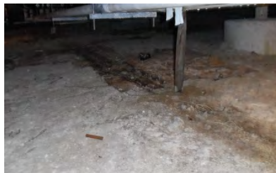
Damp soil under sweating pipes
