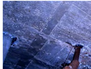
Moisture on underside of slab
