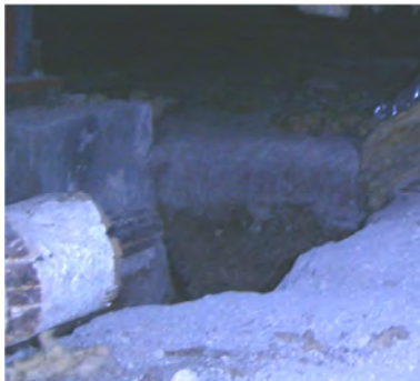
Large pit near interior pier/column
