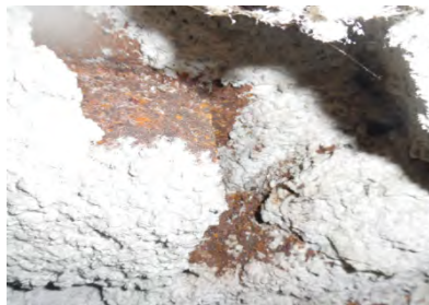
Corrosion at diagonal tube base
