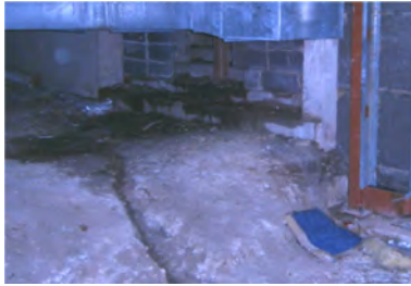
Water infiltration from abandoned staircase
