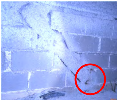
Diagonal brace with corroded base
