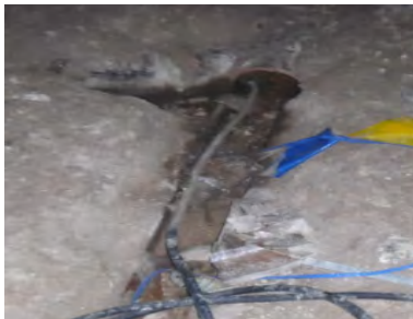
Large pipe in soil may be a drainage pipe, top of pipe is broken open for a length of roughly 10ft
